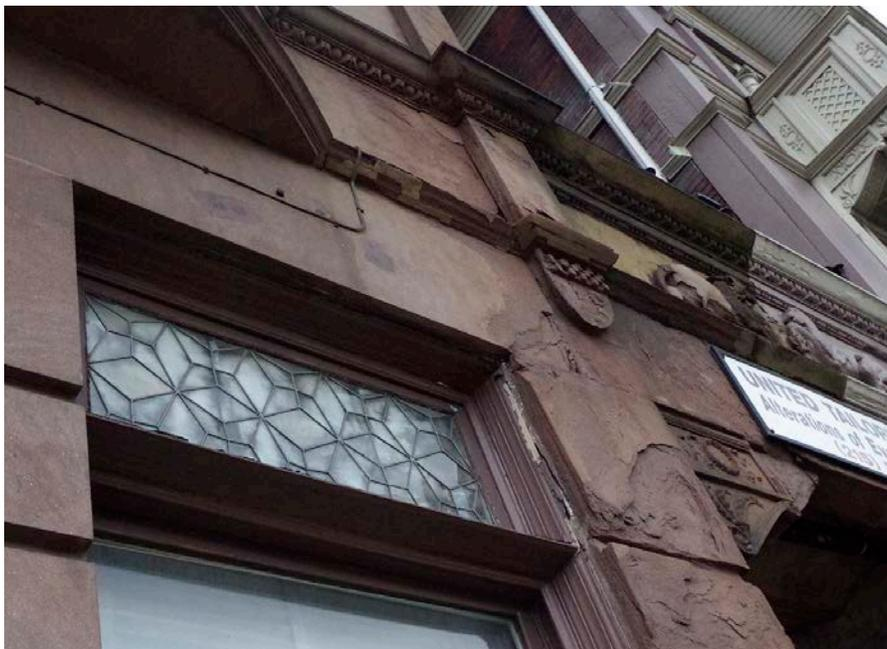
A close up of a transom window at 2305 with lead coming in a Moorish pattern and a view of the brownstone deterioration at the connecting archway. Photo: Author.
