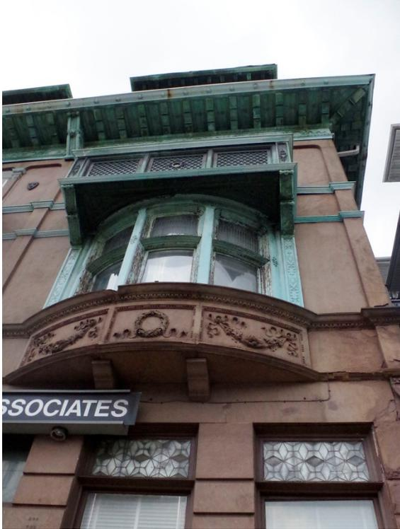
A view of the copper details at the façade of the property at 2305: an oriel window at the piano nobile, capped by a decorative balcony and a heavy, bracketed cornice below a mansard roof at the fourth floor. Photo: Author. Juliet
