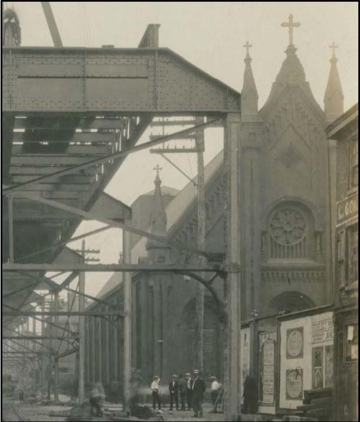
**Figure 22: “Progress of steel construction in Front St. at bent 99, looking south, June 19, 1916.” [including Immaculate Conception R.C. Church, at Allen St., two blocks bel. Girard Ave.].” Source: the Library Company of Philadelphia.**
