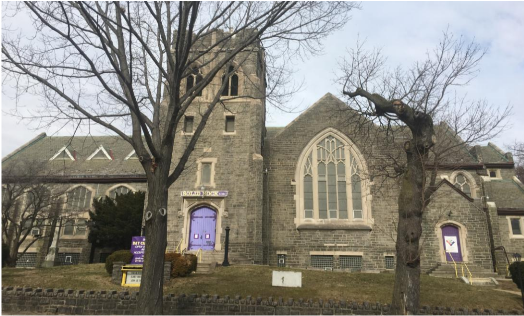
Figure 3. Looking north at the church. Photograph by Oscar Beisert.
