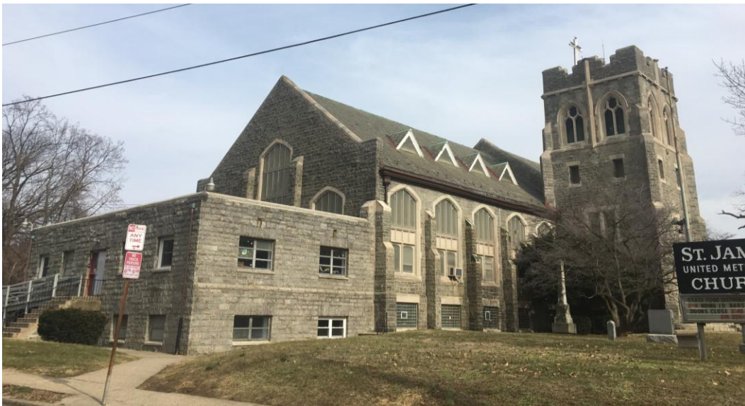
Figure 4. Looking northeast, with the 1958 addition on the left and adjoining Sunday School. Photograph by Oscar Beisert.
