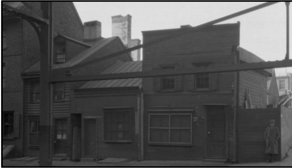
Side Gable, Double Pile Frame Vernacular Georgian Style store and dwelling (far left) and other wooden store and dwelling buildings, N. Front Street. Source: Phillyhistory.com.
