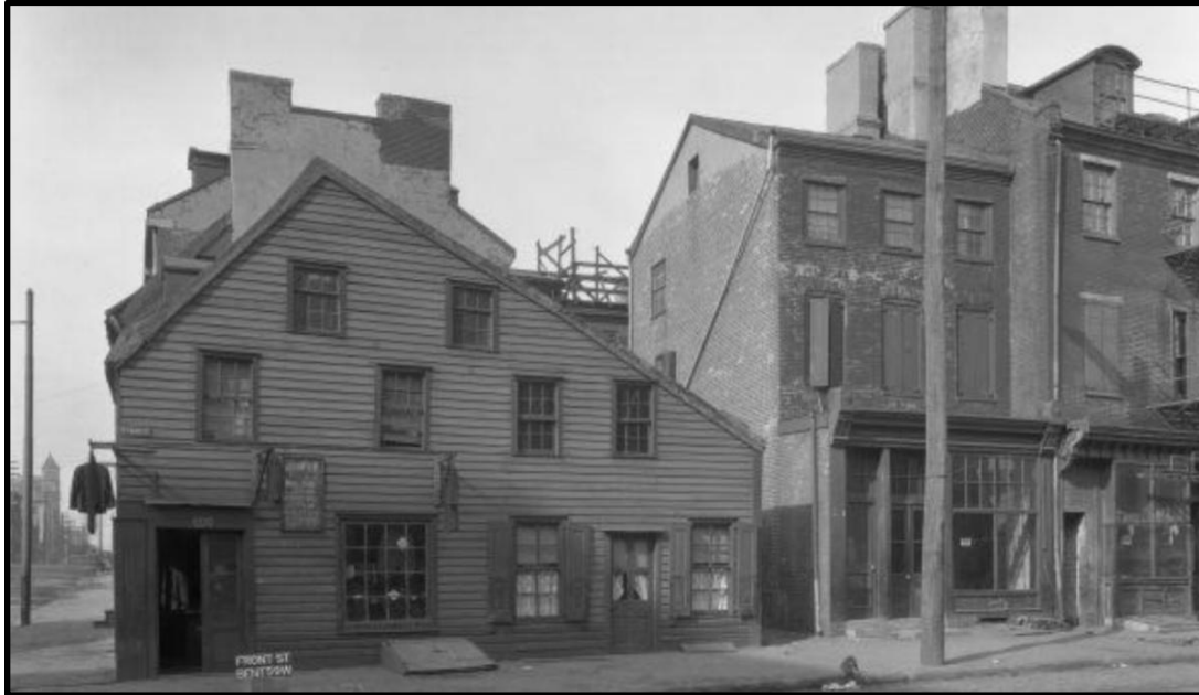
A crude version of the subject building type, a Side-Gable, Double Pile Frame Vernacular Georgian Style House, N. Front Street, Kensington. Source: Phillyhistory.com.
