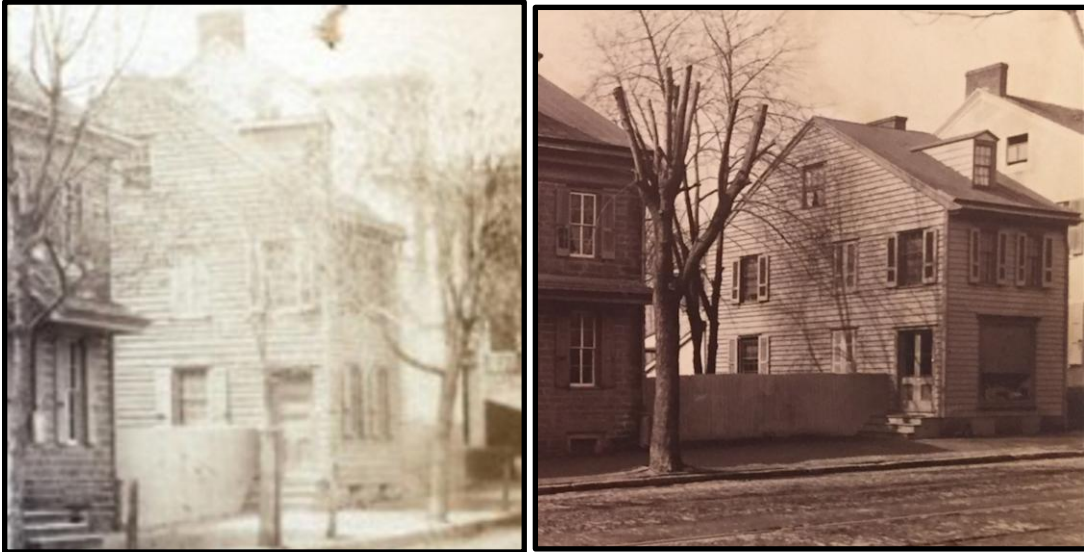
Left: frame dwelling above the Town Hall on Germantown Avenue, c. 1859. Right: the same frame dwelling post-1859. Note: the dwelling has been converted to store and dwelling, its side entrance widened and its front windows replaced with a shop window. Source: HSP.
