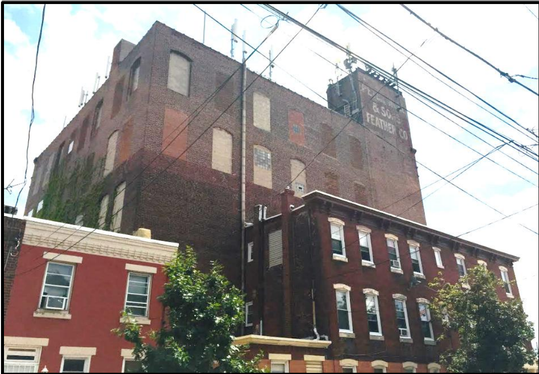
Top: Looking northeast at 173 W. Berks Street. Bottom: Looking east at the side and rear elevations of 173 W. Berks Street. Source: Oscar Beisert, 2018.
