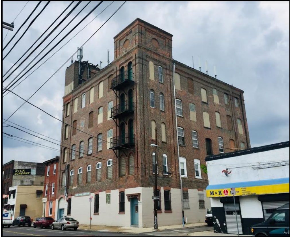
Looking northwest at 173 W. Berks Street. Source: Oscar Beisert, 2018.
