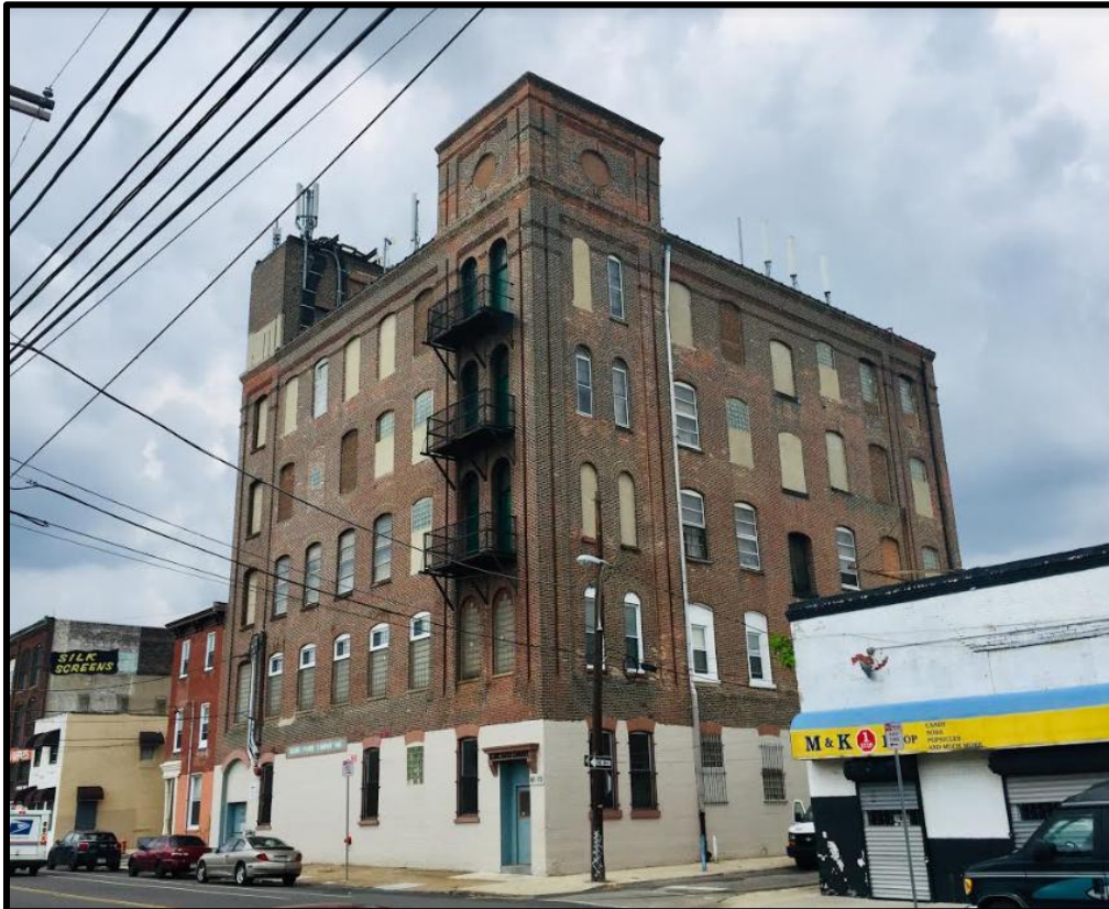
Looking south at the primary elevation of the subject property. Source: Oscar Beisert, 2018.
