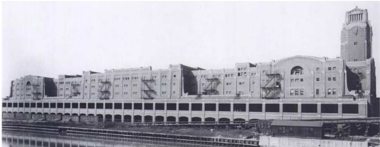
Figure 13: Chicago Freight Terminal (constructed 1914-1918) in 1918. Source: Price and McLanahan Archives, George E. Thomas Collection, from George Thomas. William L. Price: Arts and Crafts to Modern Design . (New York: Princeton Architectural Press, 2000).
