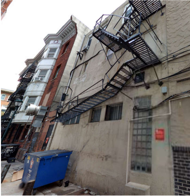
1204-06 Chancellor Street or Building 2
