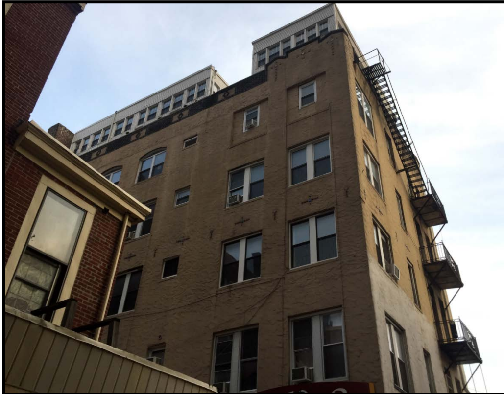
Looking southeast at the upper stories of the Camac Baths. Source: Oscar Beisert, 2018.
