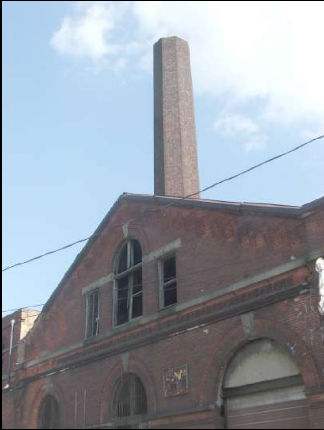
Looking southeast. Courtesy Rich Wagner.
