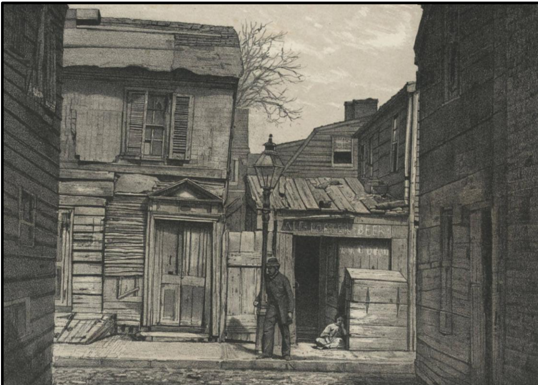
Seen between like wooden houses, the Georgian doorway in the lithograph is what remains of this like-style dwelling. In the background on right is a wooden house with a gambrel roof. This is on a whole a court of wooden houses depicted in The little homeless one or "no one to kiss me good night." Lithograph by P.S. Duval, Philadelphia, 1867. Courtesy the Library Company of Philadelphia.
