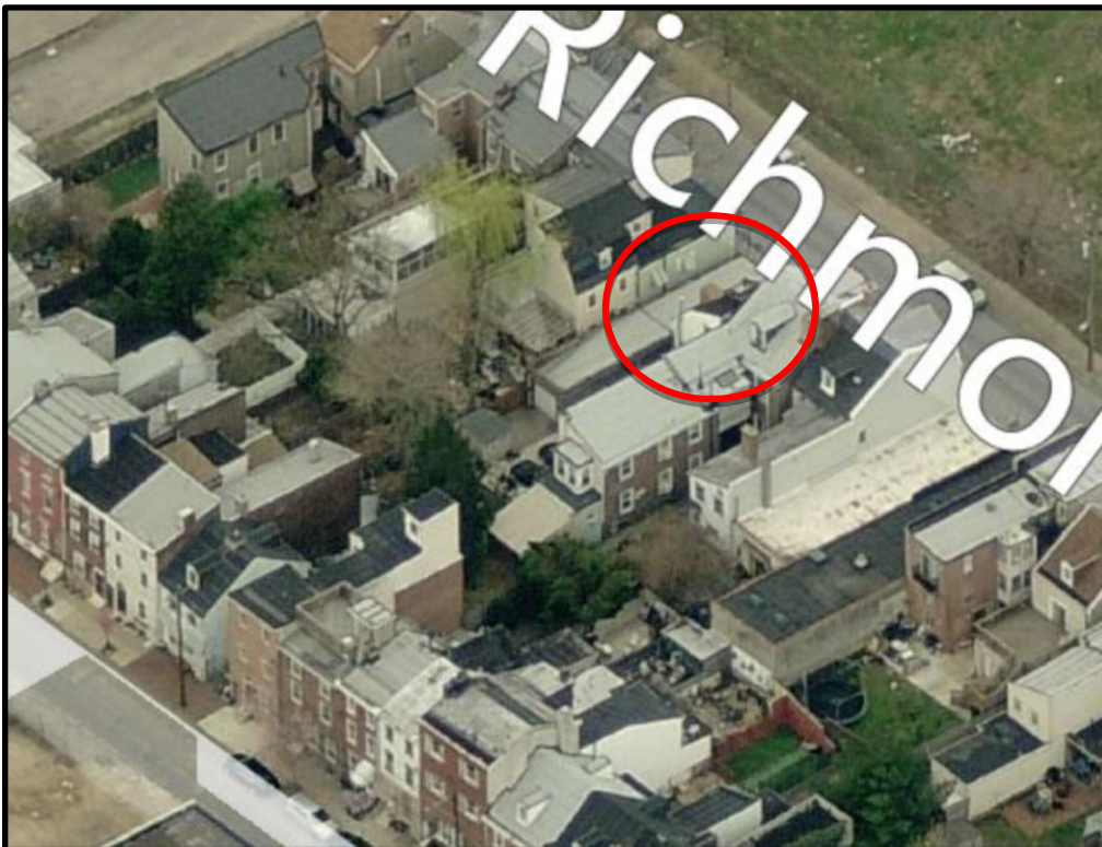
Looking southwest. Courtesy Bing Maps.
