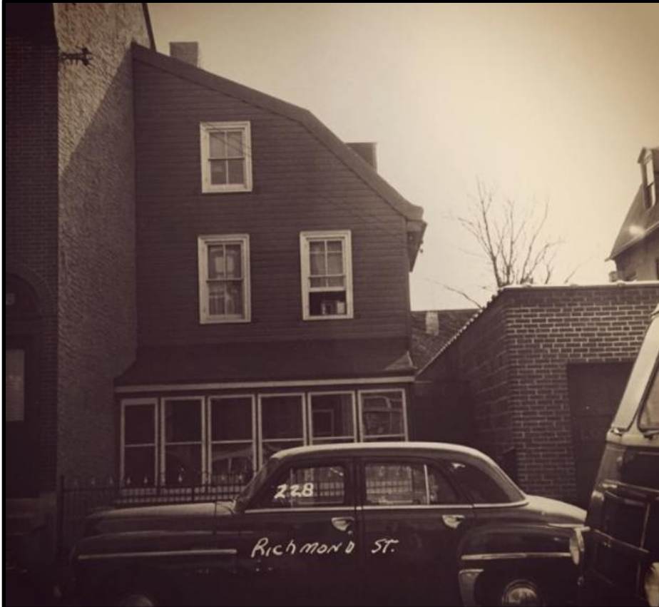
Third from the left, the Jacob Deal Half-Gambrel, Frame House appears in this photograph—then with an early version of faux siding. Taken in 1958. Courtesy the Philadelphia City Archives.
