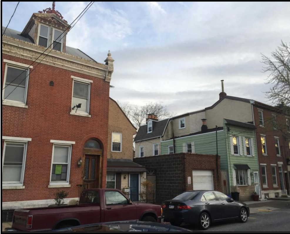
Looking southeast. Courtesy Oscar Beisert.
