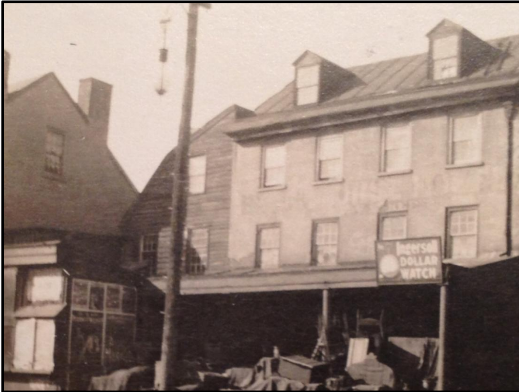
To the left of the White Horse Tavern on Frankford Avenue is a gable-front House with the broken pitch, gambrel style roof. Courtesy the Historical Society of Pennsylvania.
