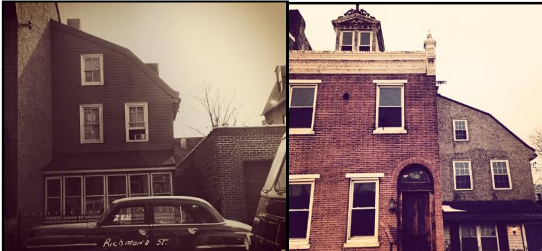
Left: Wooden Half-Gambrel, Gable-Front House at 228 Richmond Street. Note the single dormer projecting to the side of the lot and that a house at the same recessed position is peaking out on right. Courtesy the City of Philadelphia. Right: Extant Wooden Half-Gambrel, Gable-Fronted House at 228 Richmond Street. Note the same building appears on left to-date. Photography by Oscar Beisert.
