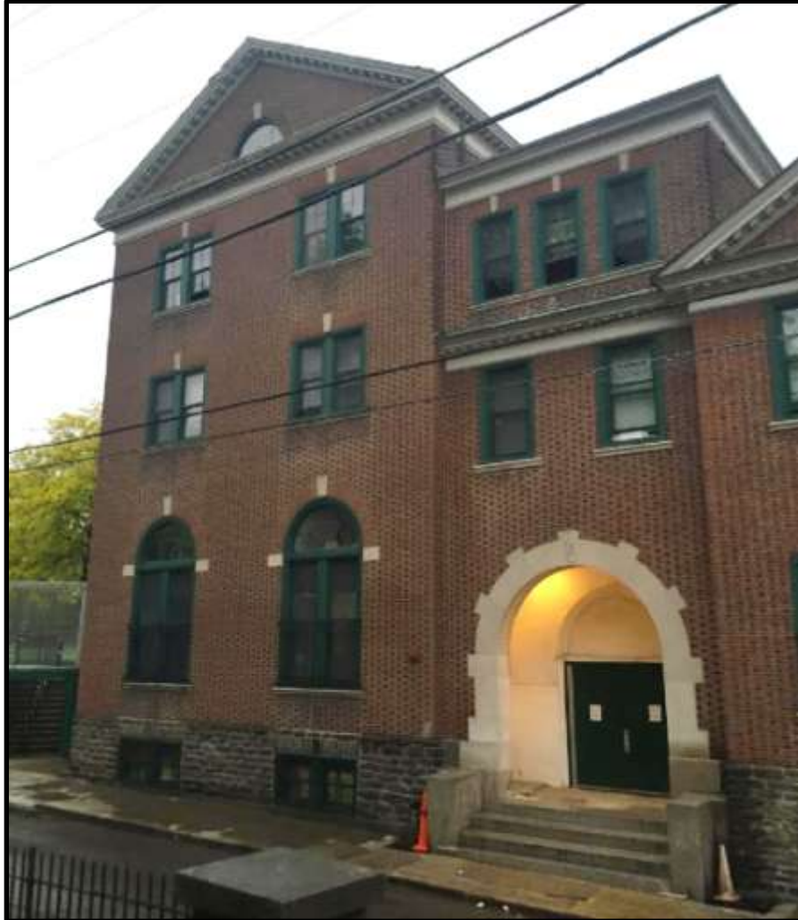
Looking southwest, the 1909 Addition. Photograph by Oscar Beisert.
