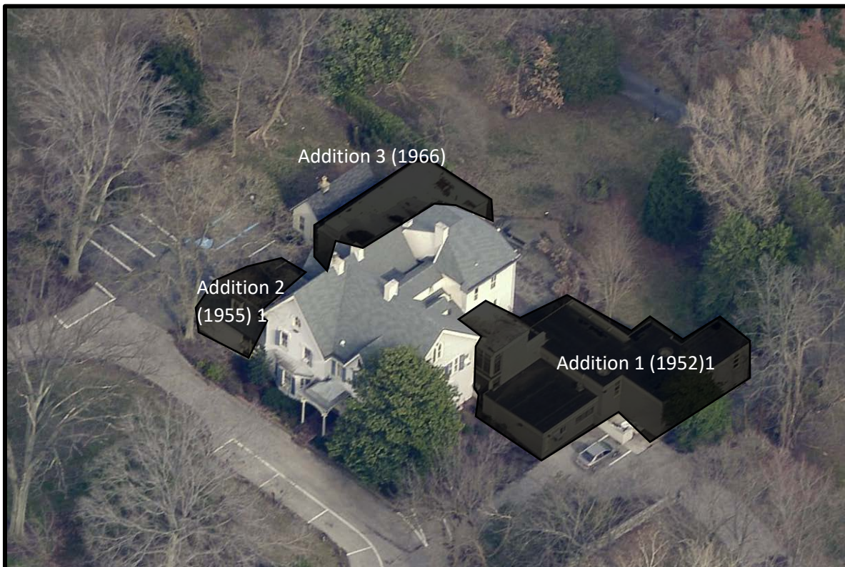
Figure 14. Looking northeast at the subject property, the non-contributing portion is highlighted in black—Additions 1, 2, and 3. Source: Atlas, City of Philadelphia, 2018.
