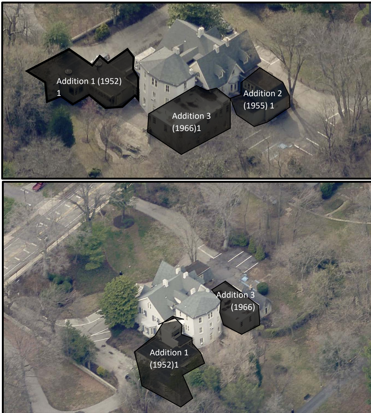
Figure 15. Top: Looking southwest at the rear of the subject property, the non-contributing portions are highlighted in black—Additions 1, 2 and 3. Bottom: Looking northwest at the rear elevation of the property, the non-contributing portions are highlighted in black—Additions 1 and 3. Source: Philadelphia Atlas.
