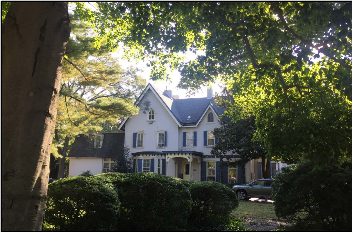
Figure 3. Top: The primary (northwest) elevation and yard of the subject property. Bottom: The primary (northwest) elevation of the subject property. Source: Oscar Beisert, 2018.
