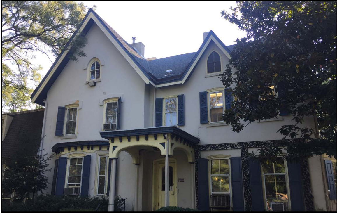
Figure 4. The primary (northwest) elevation. Source: Oscar Beisert, 2018.
