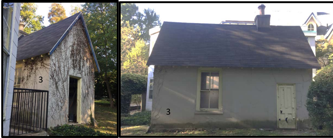
Figure 13. The numbers used in the photographs above correspond with the list of “Landscape Features” at the center of the previous page. Left: Looking northwest at the rear elevation of the shed building in the Gothic Revival style. Right: Looking south at the side (northeast) elevation of the shed building. Source: Oscar Beisert, 2018.
