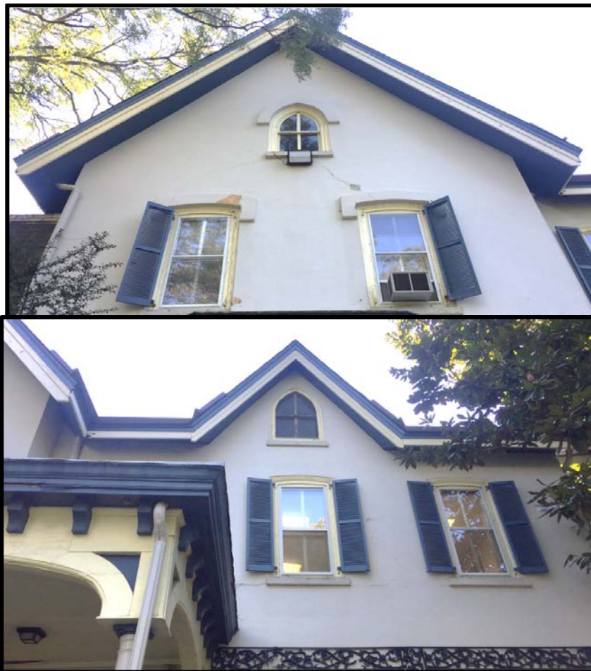
Figure 5. Top: The upper floors of the larger gable end within the primary (northwest) elevation of the subject property. Note, the window, defined by the pointed arch, as well as the window hoods on both floors. Bottom: The smaller gable within the primary (northwest) elevation. Source: Oscar Beisert, 2018.
