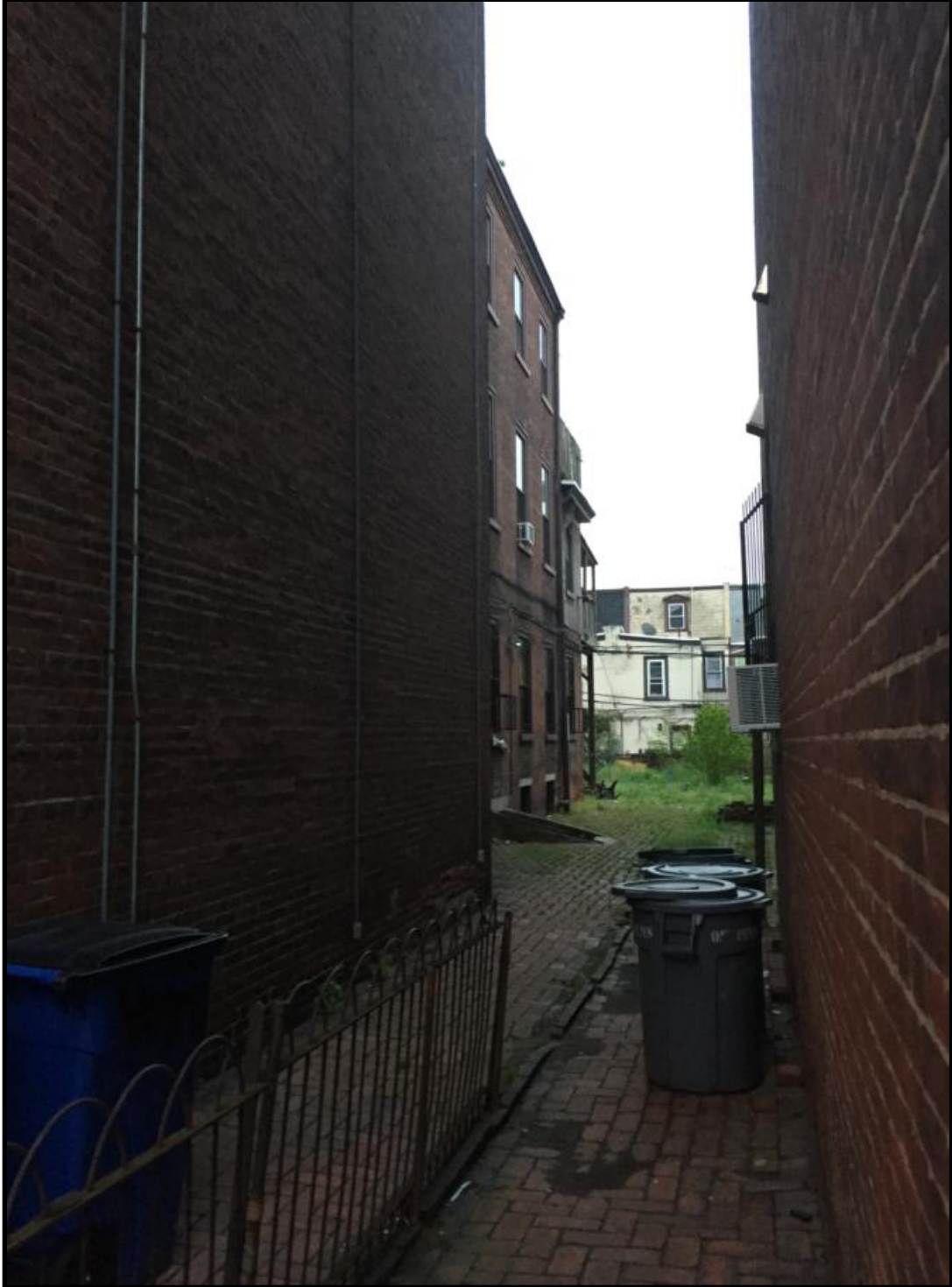
Looking south at the rear elevation of 4050 Chestnut Street. Courtesy Oscar Beisert.
