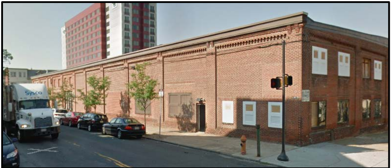
Looking southwest at Building No. 3. Source: Google Earth.
