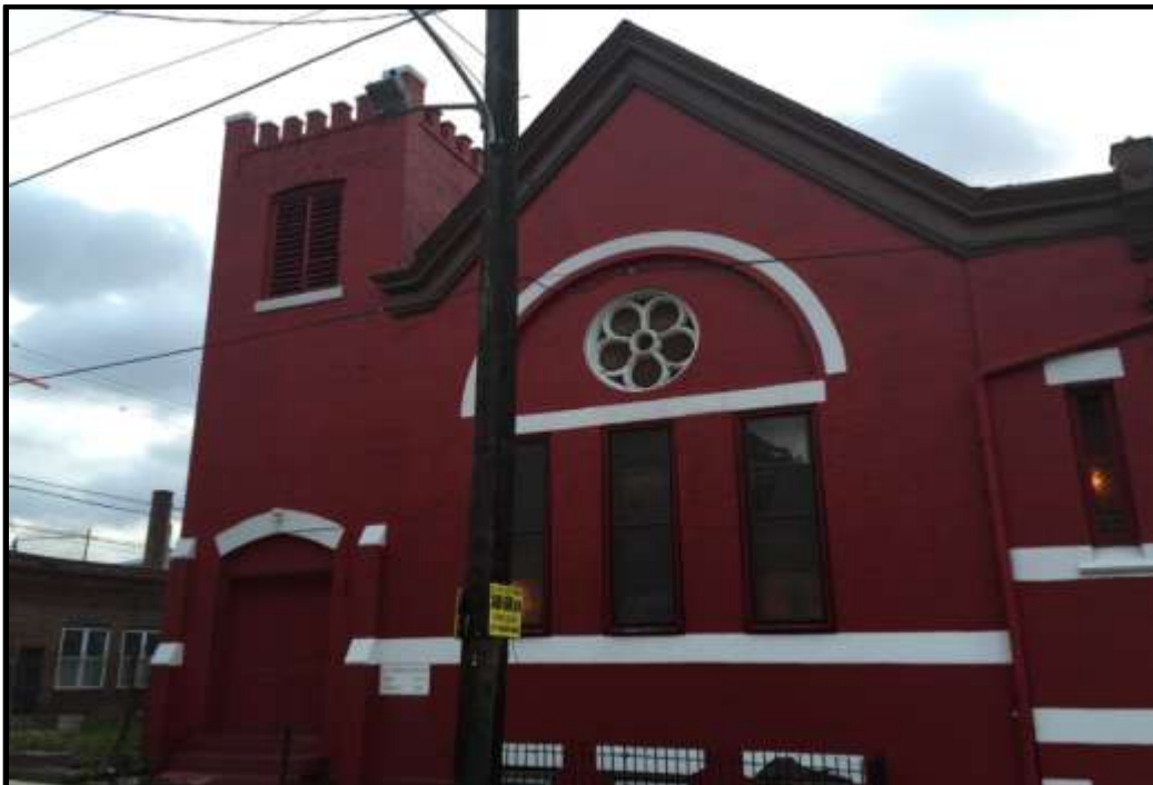
Looking southwest. Courtesy Oscar Beisert.
