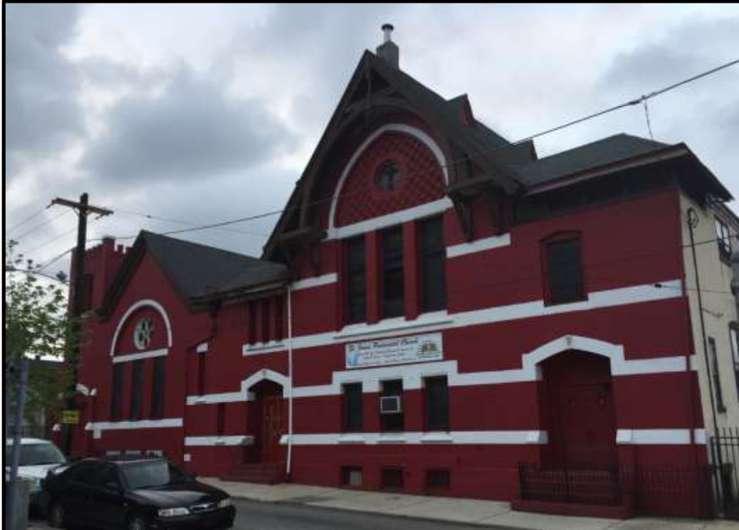
Looking southwest. Courtesy Oscar Beisert.
