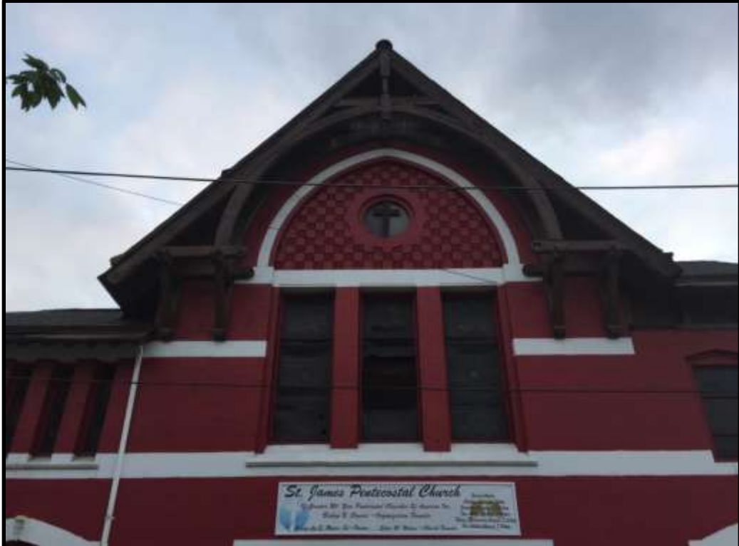
Looking west at the gable of the 1884 Addition. Courtesy Oscar Beisert.
