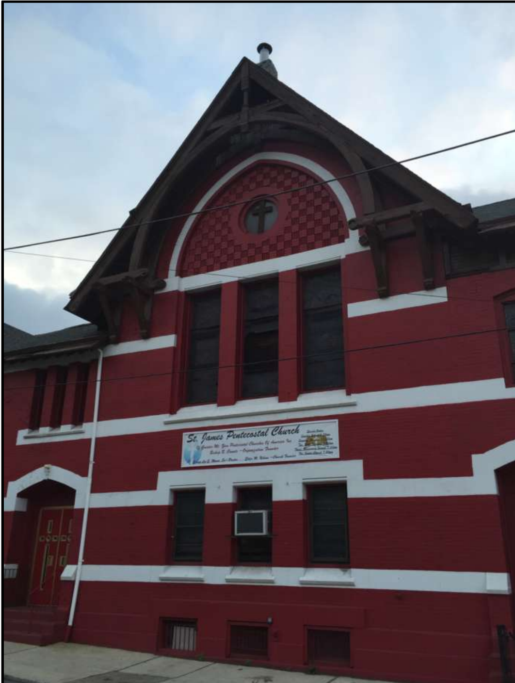
Looking southwest. Courtesy Oscar Beisert.
