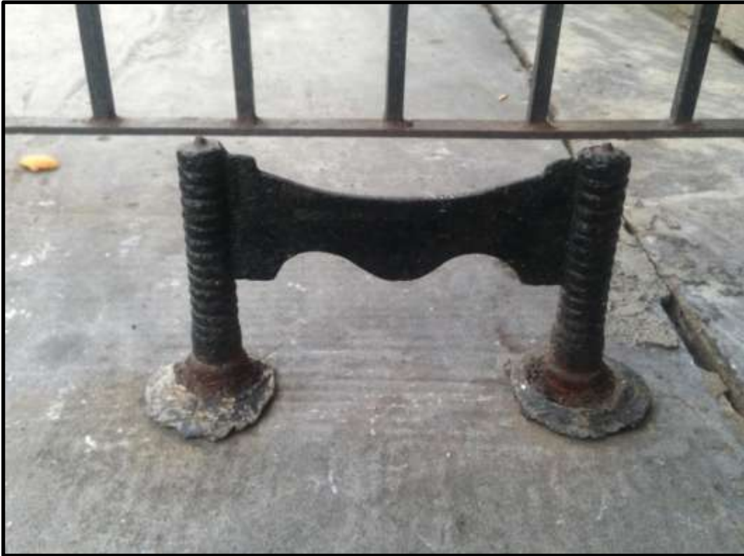
Looking at a detail of the iron boot scraper set upon the marble base of the entrance porch. Courtesy Oscar Beisert.
