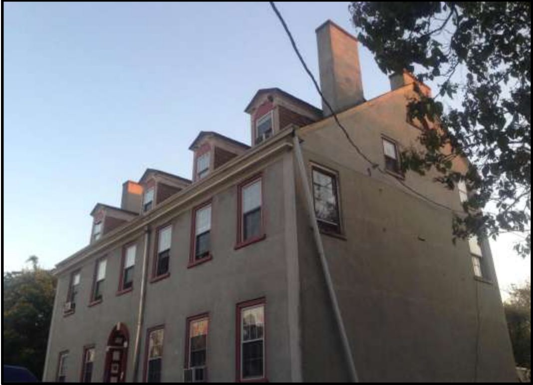
Looking southeast. Courtesy Oscar Beisert.
