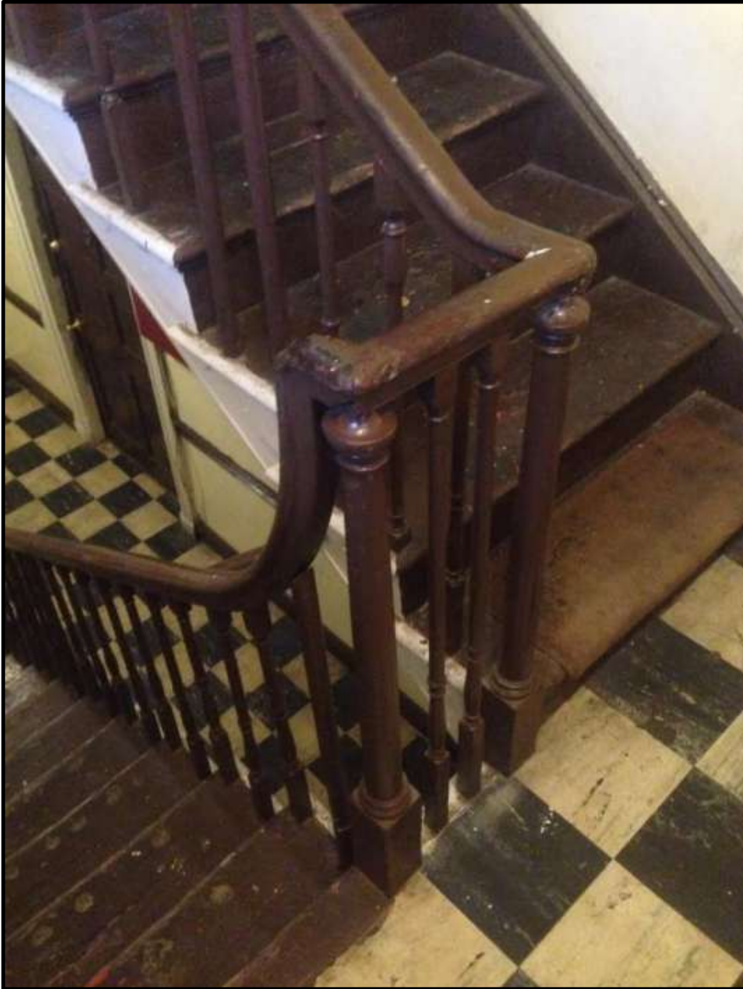
Federal period staircase details. Courtesy Oscar Beisert.
