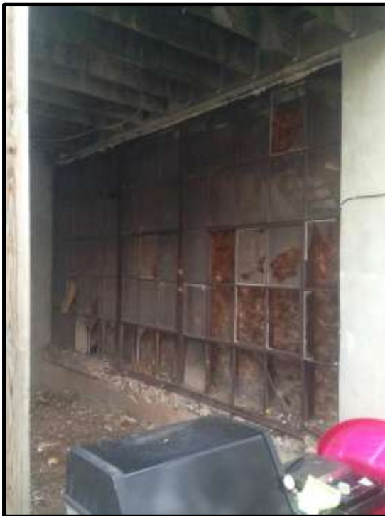
Looking northwest at a multi-light industrial metal window within the stable. Courtesy Oscar Beisert.
