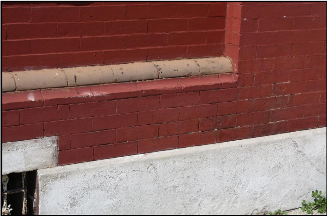
Looking north. Within the recessions created by the ornamental brickwork are spans of bull nosed brick. Courtesy Janette Amstutz.
