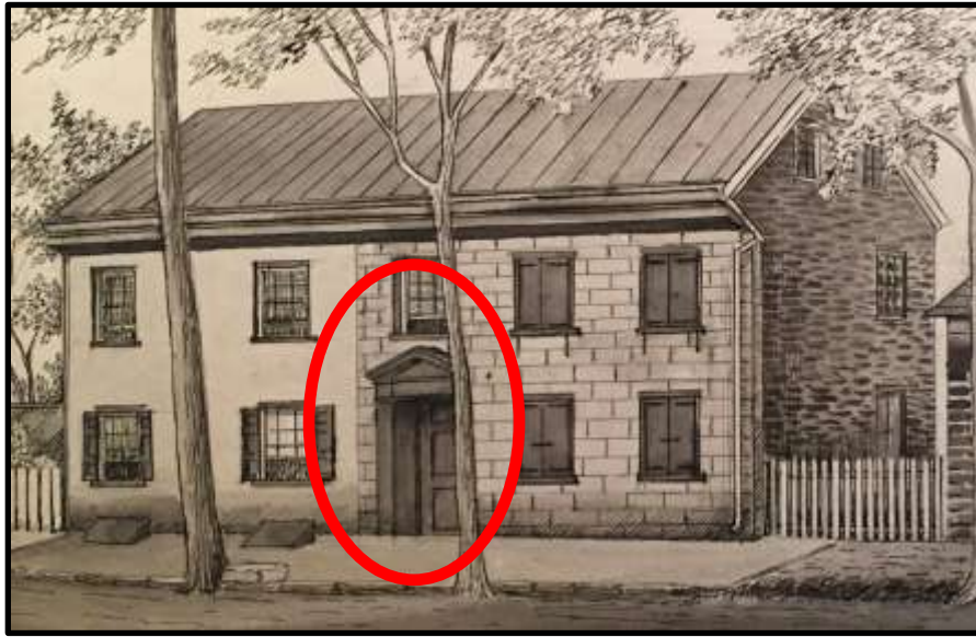
The drawing above is of a farmhouse owned at one time by Christopher Ludwig, then the Baker General. The house was once located on Haines Street. Like the subject house, it may have grown over time to suit the needs of the owner. It too features certain Georgian stylistic details such as the architrave and pediment. Taken from Old Landmarks of Germantown and Vicinity by John Richard. Courtesy the Historical Society of Pennsylvania.
