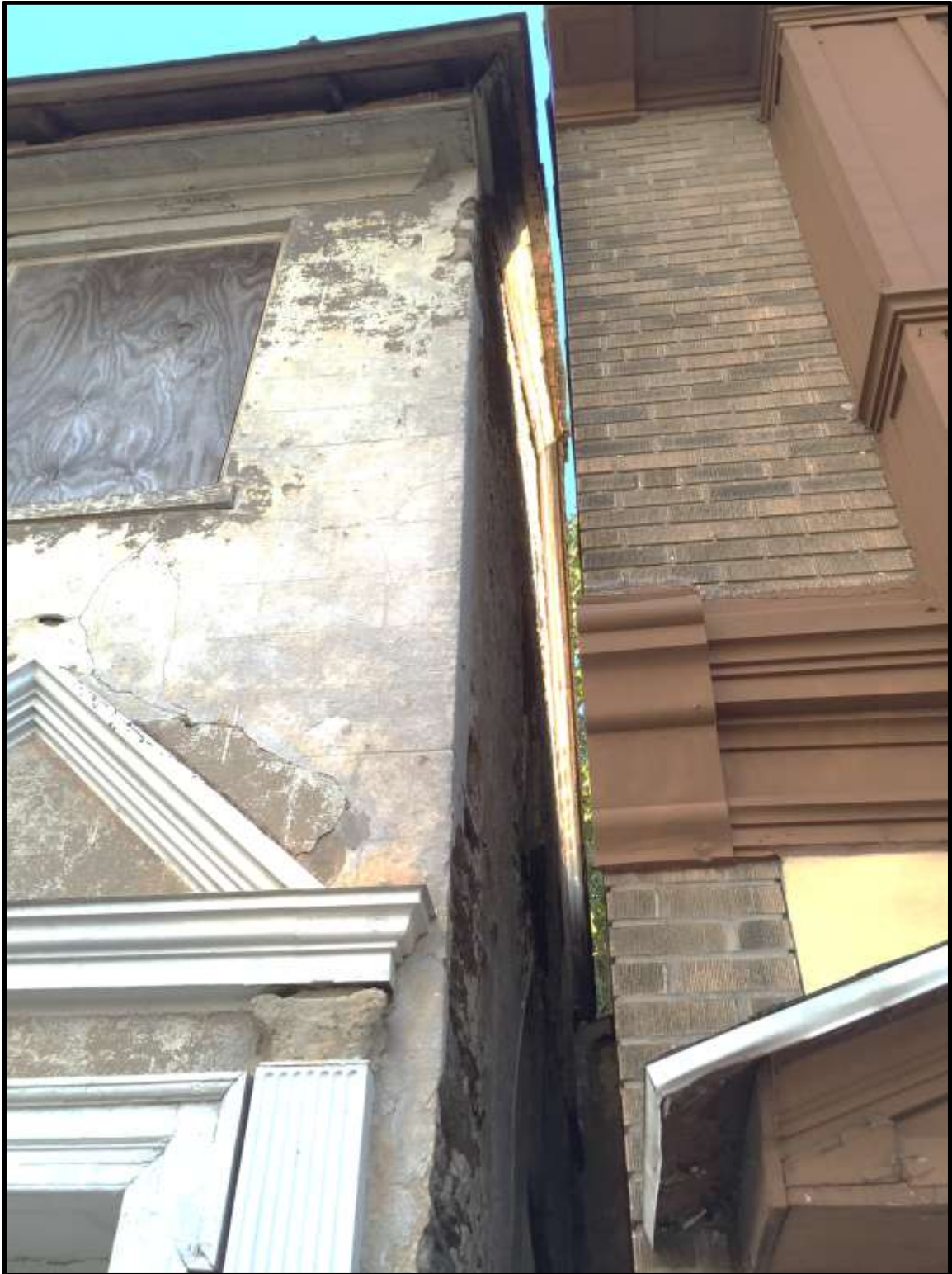
Looking southwest. Courtesy Oscar Beisert.
