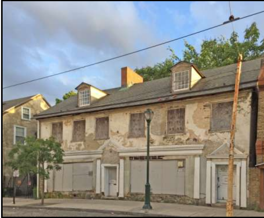
Looking southwest. Courtesy Oscar Beisert.
