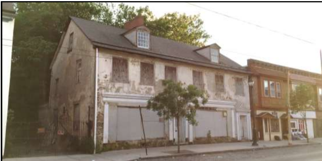
Looking southwest. Courtesy Oscar Beisert.
