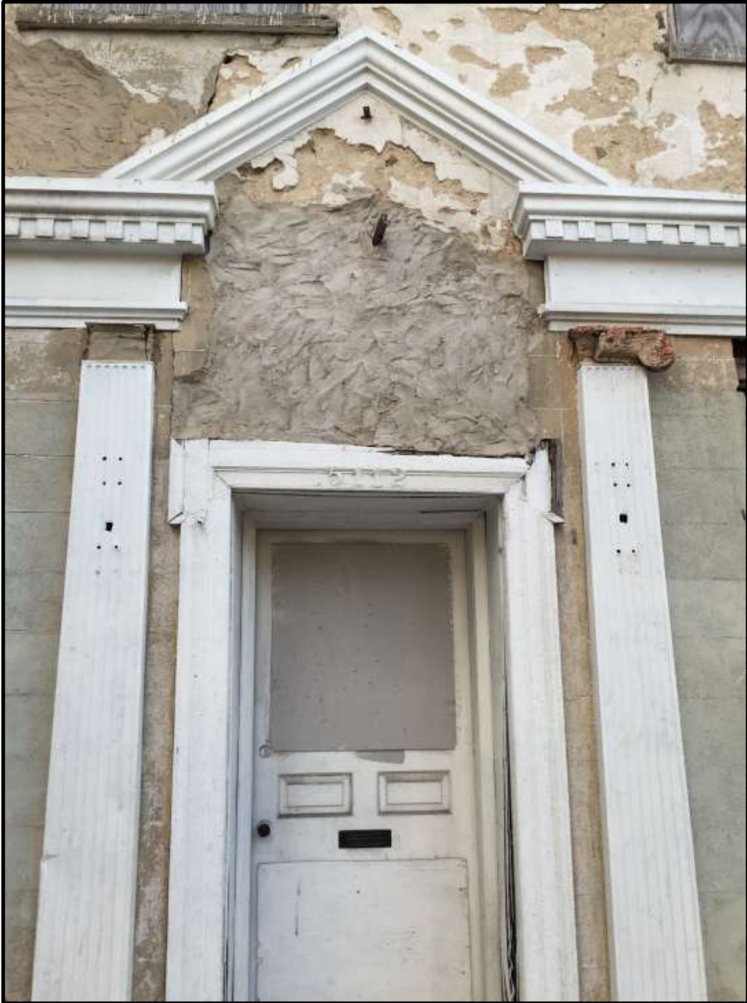
Looking southwest. Courtesy Oscar Beisert.
