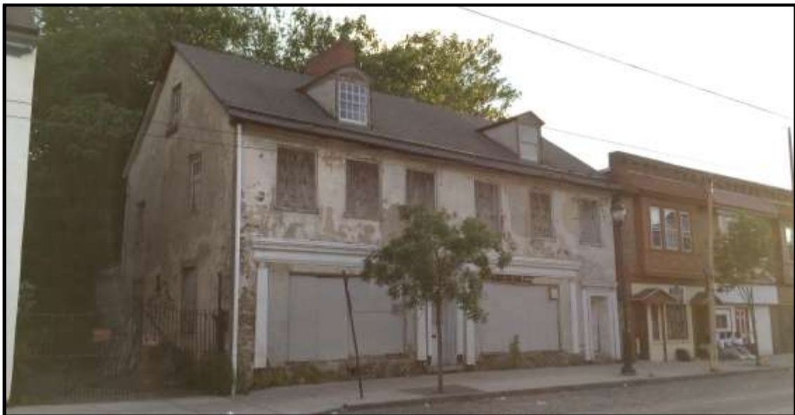
Looking southwest. Courtesy Oscar Beisert.
