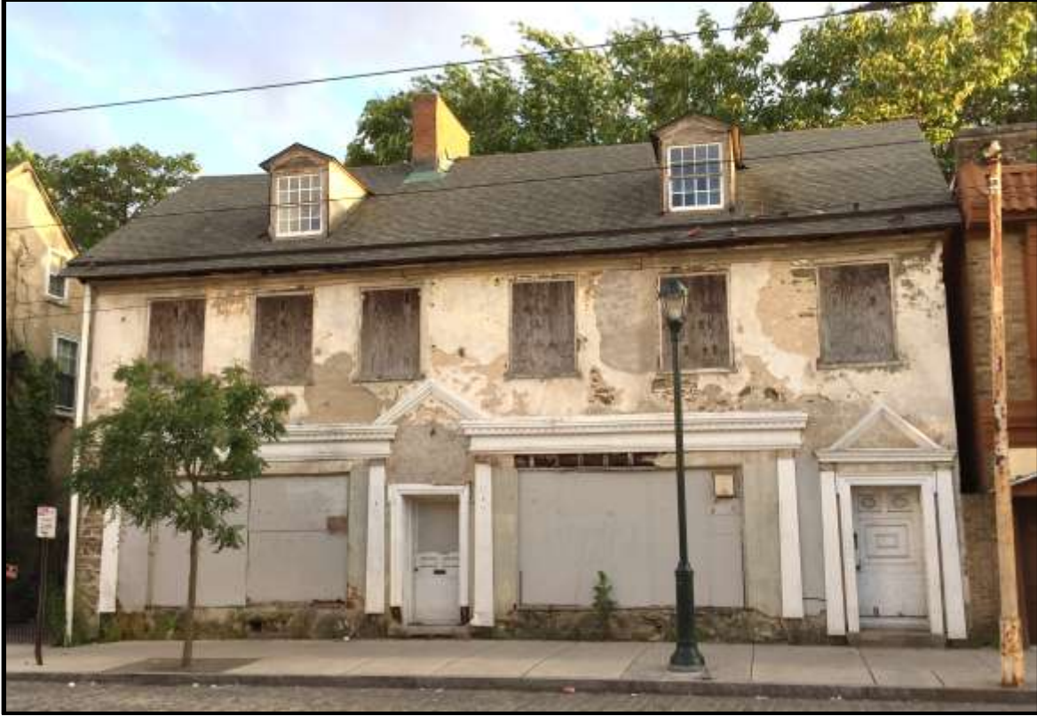
Looking southwest. Courtesy Oscar Beisert.
