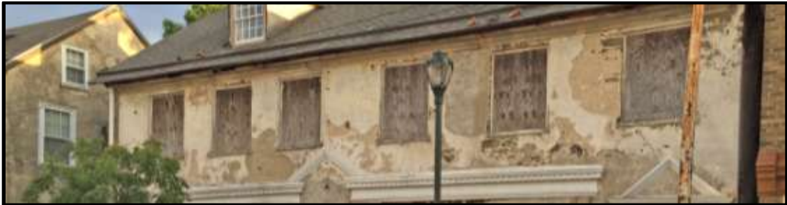
Looking southwest. Courtesy Oscar Beisert.
