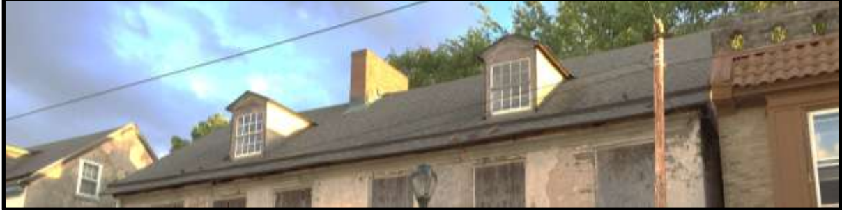
Looking southwest. Courtesy Oscar Beisert.
