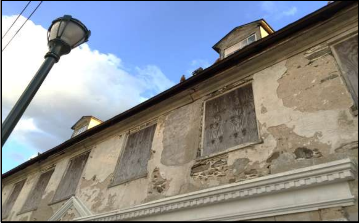
Looking southwest. Courtesy Oscar Beisert.
