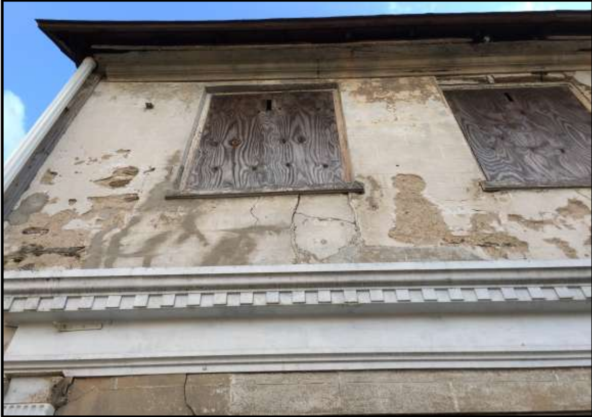
Looking southwest. Courtesy Oscar Beisert.
