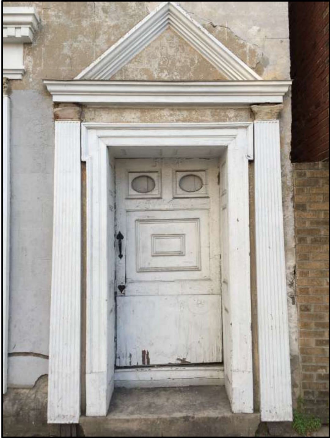
Looking southwest. Courtesy Oscar Beisert.
