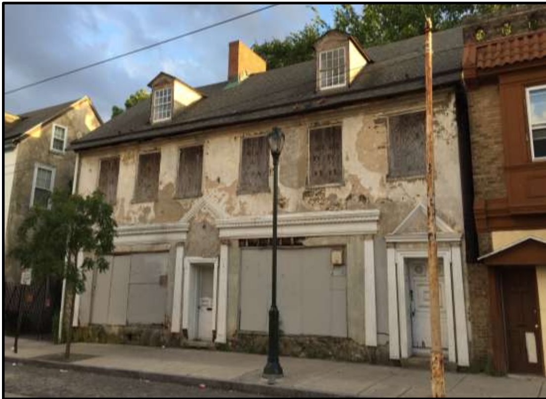
Looking southwest. Courtesy Oscar Beisert.
