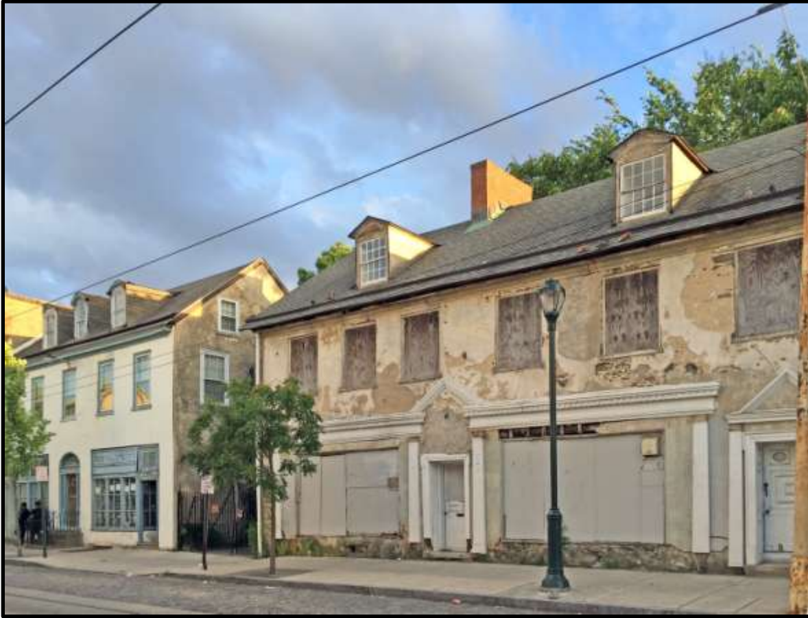
Looking southwest. Courtesy Oscar Beisert.
