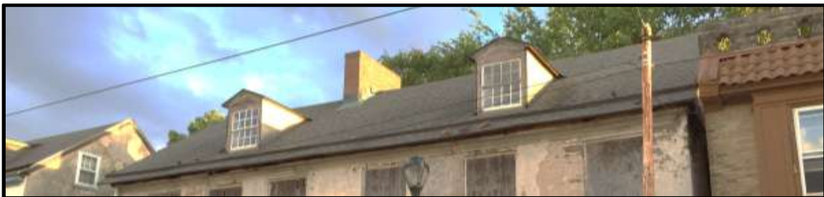
Looking southwest. Courtesy Oscar Beisert.
