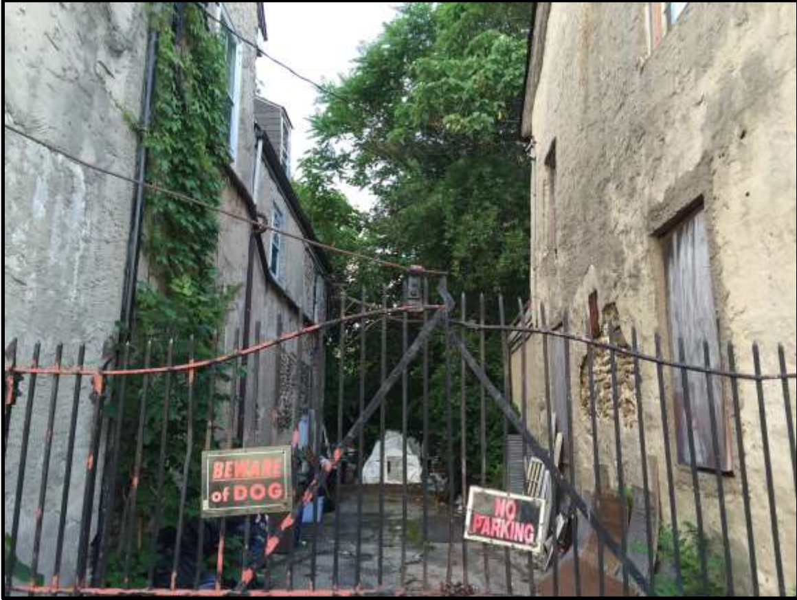
Looking southwest. Courtesy Oscar Beisert.
