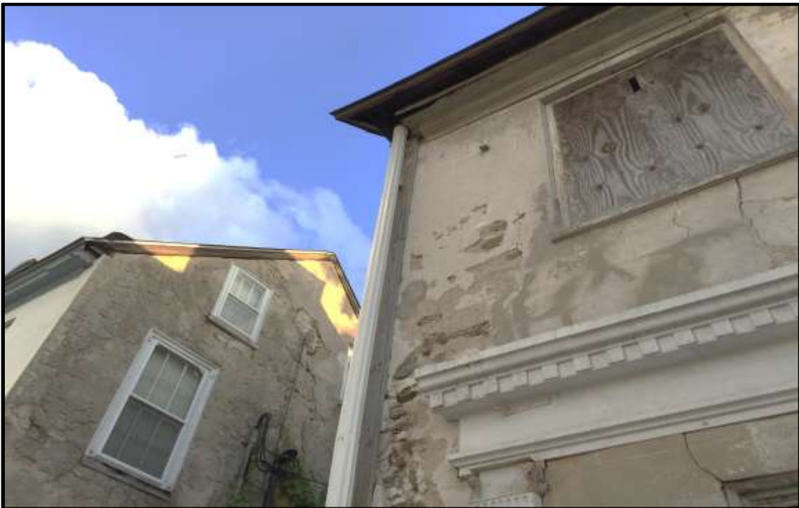
Looking southwest. Courtesy Oscar Beisert.
