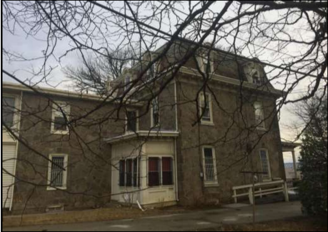
Looking northwest. Courtesy Oscar Beisert.
