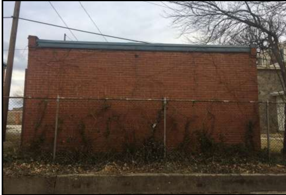
Looking northwest. Courtesy Oscar Beisert.
