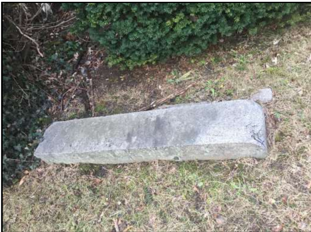
Granite post at the east corner of the property along Chew Avenue. Courtesy Oscar Beisert.
