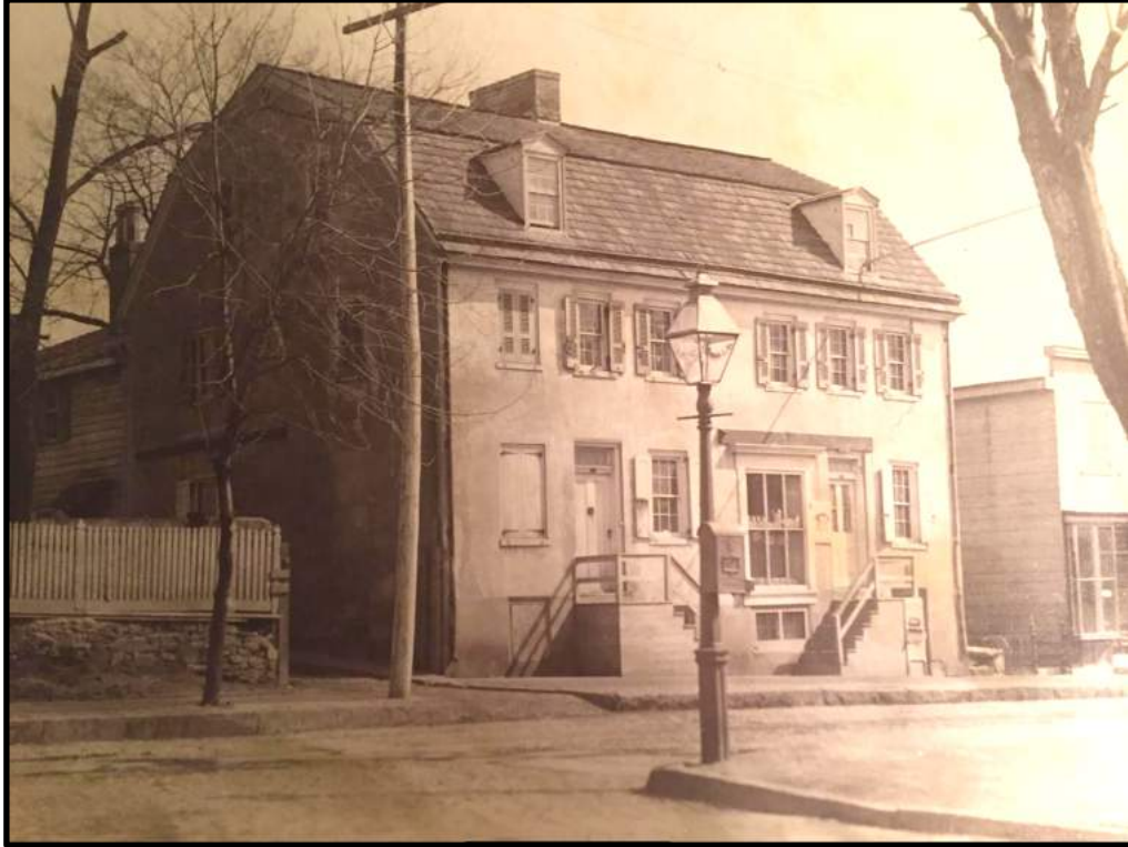
Situated on Germantown Avenue opposite Tulpehocken Street, the Store and Dwelling of Henry Freas, c. 1890. On right is another store building, which was of wood frame construction. This is clearly an eighteenth century house that was altered to accommodate a store; however, the subject conversion may be an early example. Demolished 1913. Source: the Historical Society of Pennsylvania.
