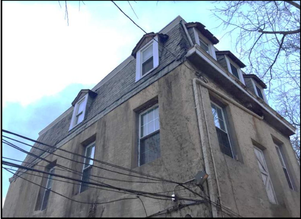
Looking northwest. Courtesy Oscar Beisert.
