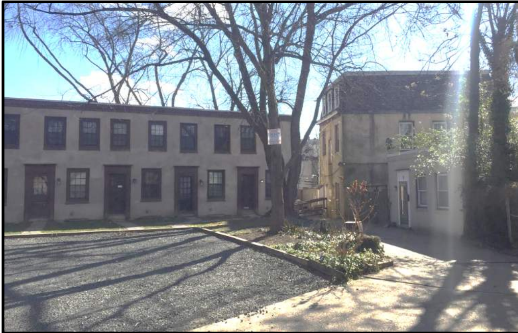
Looking south into Harrison Court. Courtesy Oscar Beisert.
