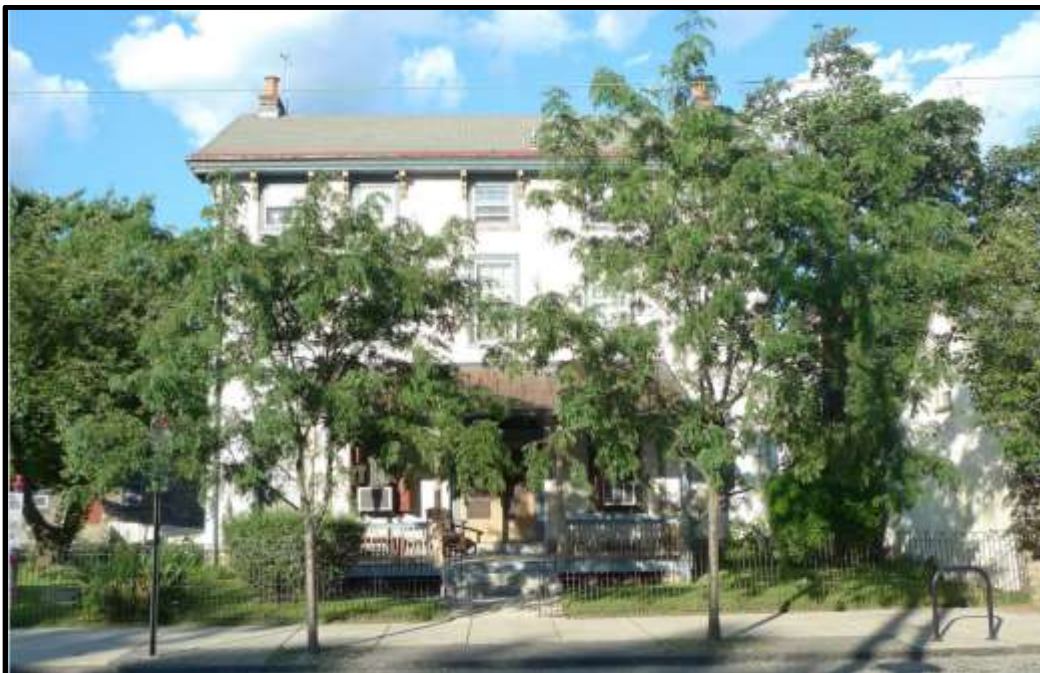
The primary elevation of the Parsonage facing Germantown Avenue. Source: J.M. Duffin.
