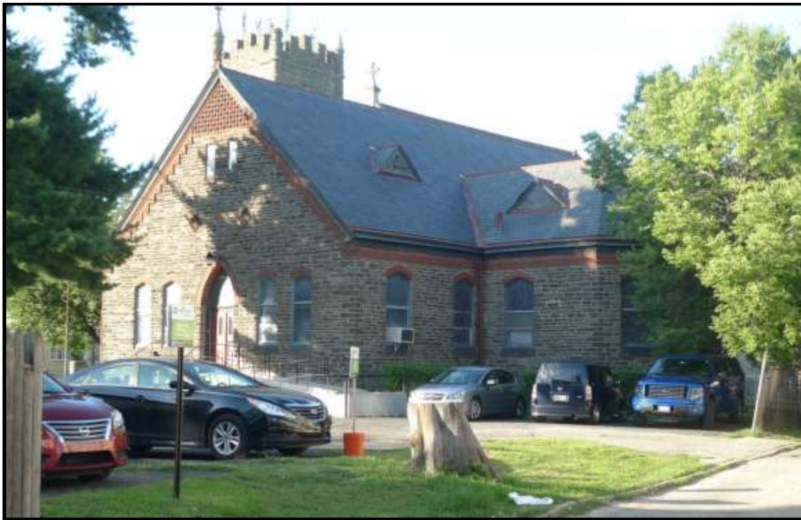
The southwest and southeast elevations of the Sunday School. Source: J.M. Duffin.
