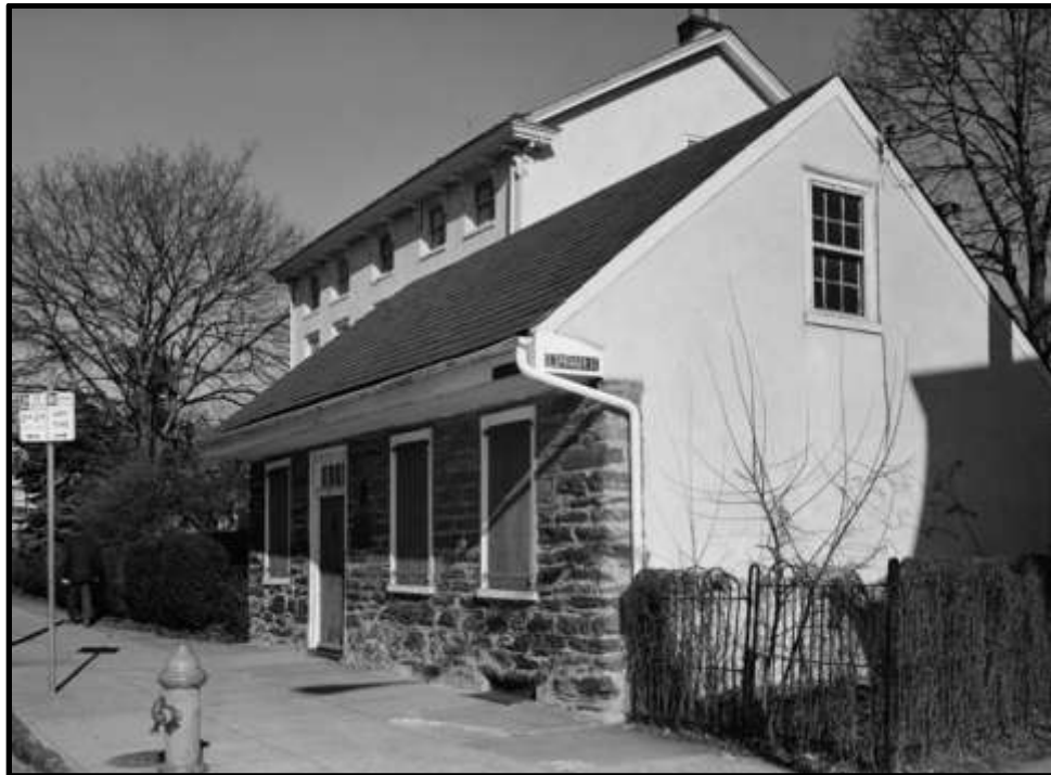
Primary elevation along the Germantown Avenue right-of-way. Currently occupied by a bakery. Source: https://en.wikipedia.org/wiki/Beggarstown_School#/media/File:Beggarstown_School.jpeg
