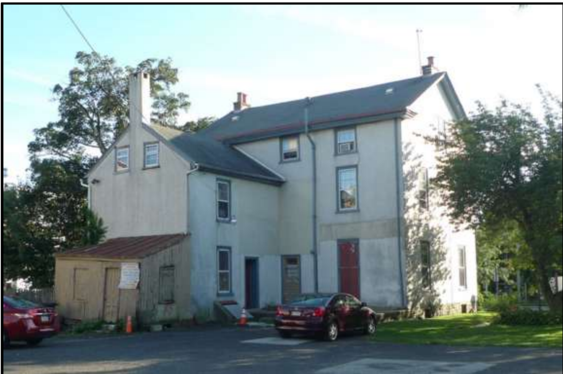
The rear of the Parsonage showing the different volumes. Source: J.M. Duffin.
