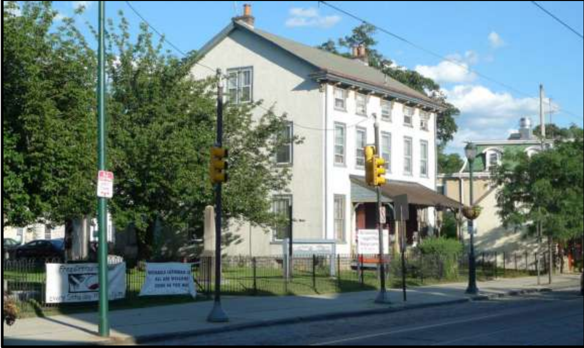
The southwest elevation of the Parsonage showing the side gable. Source: J.M. Duffin.
