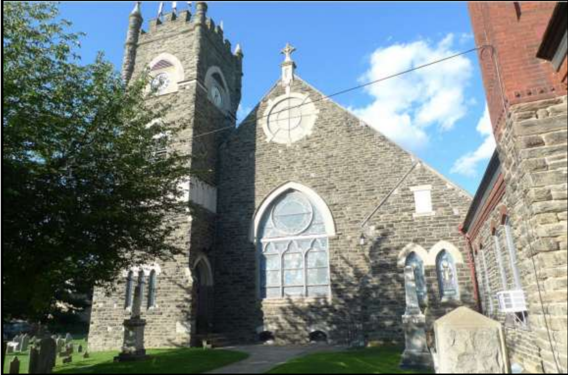
The southwest and primary elevation of the Church. Source: J.M. Duffin.
