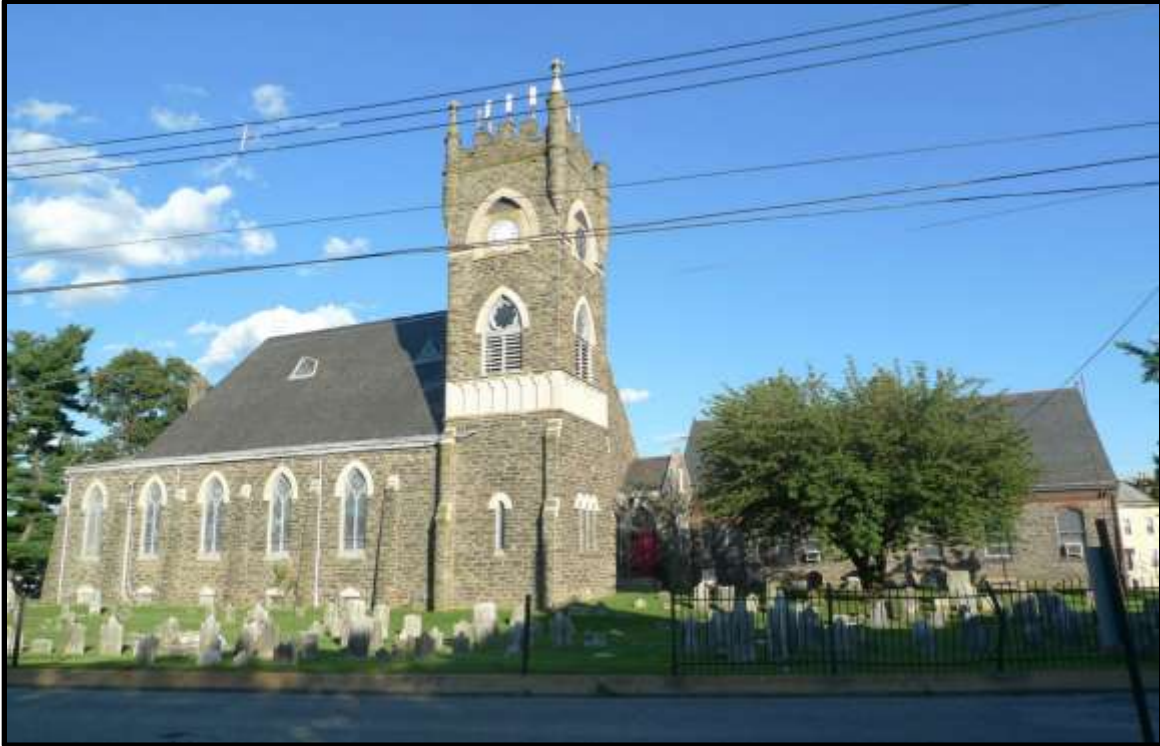
The northwest elevation of the Church. Source: J.M. Duffin.
