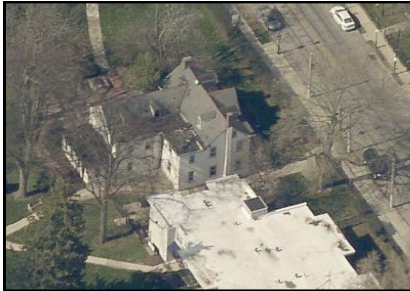
Looking north at the rear wing, the rear additions, and the main block. Source: Pictometry, City of Philadelphia.
