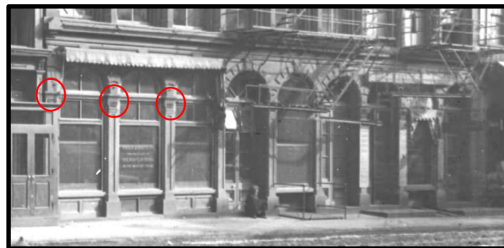
Figure 21: Philadelphia Quartz Company's building at 121 3rd Street, Philadelphia, showing pilasters with similarly stylized capitals. Source: Hagley Digital Archives
