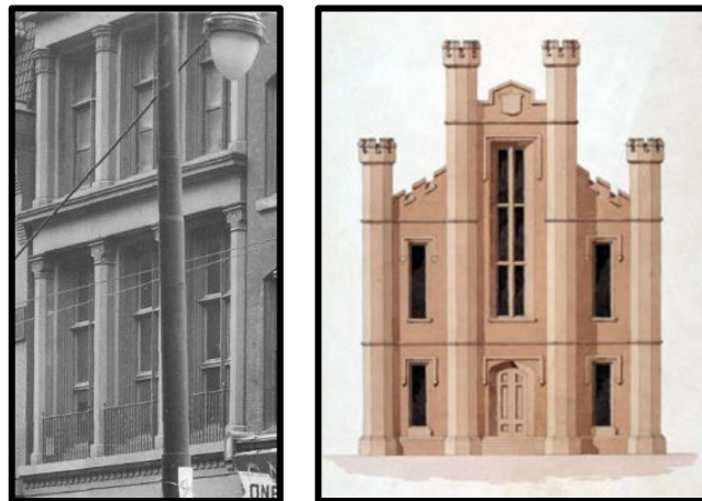
Figure 16: Left: A detail of the octagonal pilasters that define the primary (north) elevation of the subject property Source: Chestnut Street—700 Block (NE corner 8 th and Chestnut), City of Philadelphia Records Department. Right: Design for the Pennsylvania Medical College, 9 th Street below Locust, c. 1849, by Thomas Ustick Walter, which employs octagonal towers and/or pilasters in its primary elevation. Source: The Athenaeum of Philadelphia.
