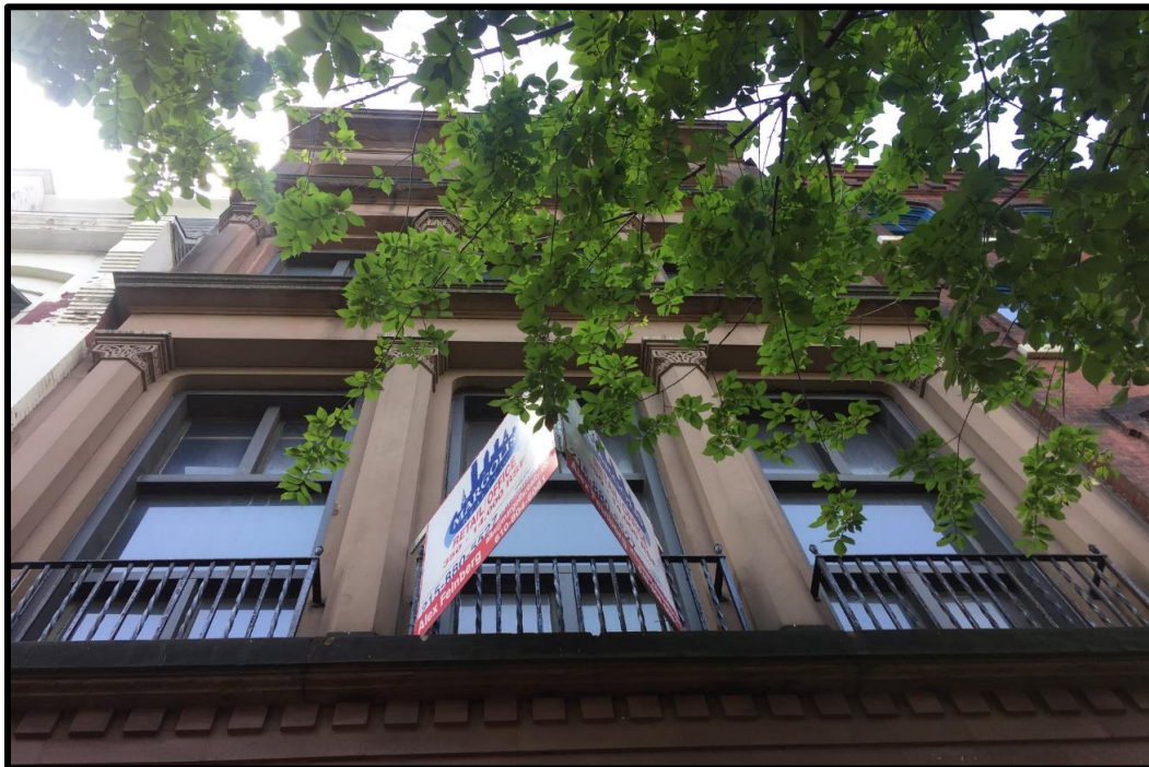
Figure 6: Top: Chestnut Street—700 Block (NE corner 8 th and Chestnut). Source: City of Philadelphia Records Department. Bottom: Looking upward at the primary (north) elevation of 726 Chestnut Street. Source: Oscar Beisert.
