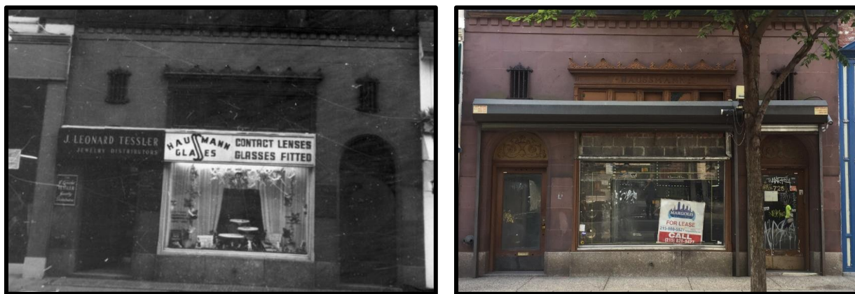
Figure 26: Left: The storefront of the primary (north) elevation, c. 1960-70. Source: Philadelphia Historical Commission. Right: the same view in 2018. Source: Oscar Beisert.
