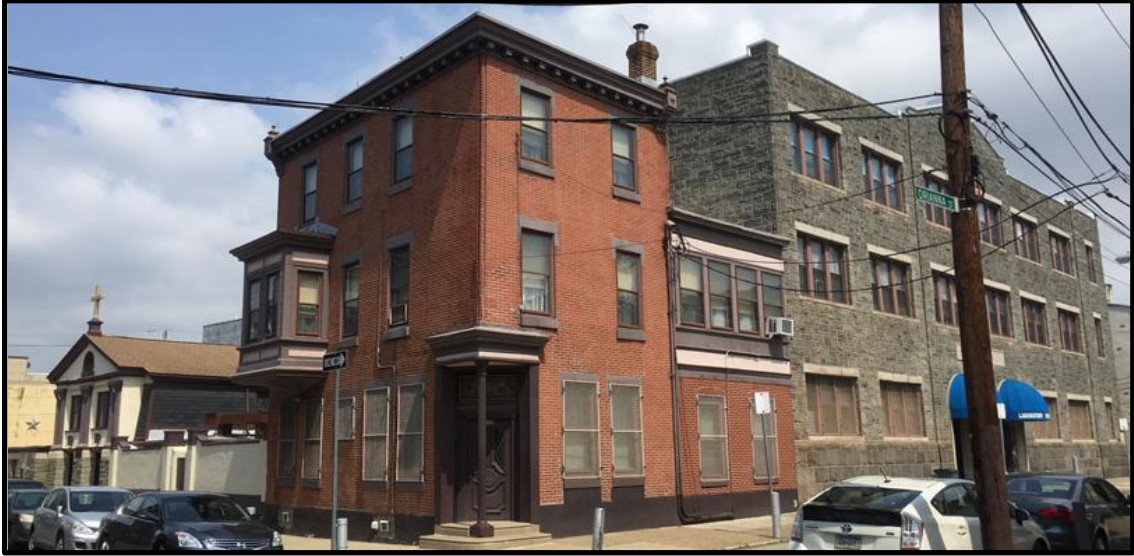
Looking northwest at the church (on left), the rectory (at center), and the school (on right) of St. Agnes. Source: Oscar Beisert.
