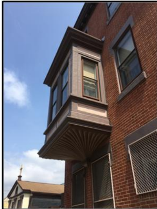
Looking northwest, a bay window of the Rectory. Source: Oscar Beisert.
