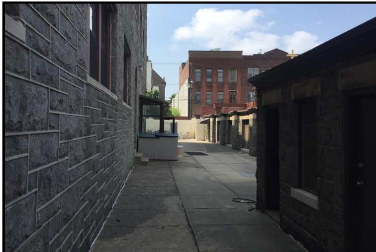
Looking south at the interior court of the buildings of St. Agnes. Source: Oscar Beisert.
