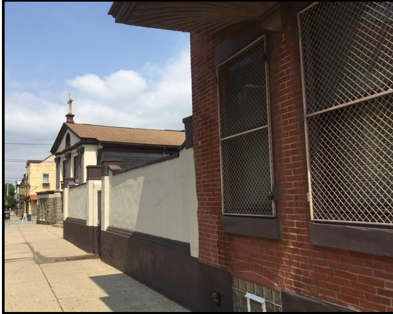
Looking northwest, the ground floor of the rectory, a high brick wall, and the church in the distance. Source: Oscar Beisert.
