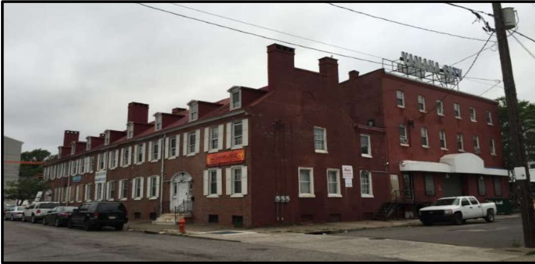
Looking northwest. 81–95 Fairmount Avenue (left) and the Wagon House of J. Campbell Harris & Co. (right)
