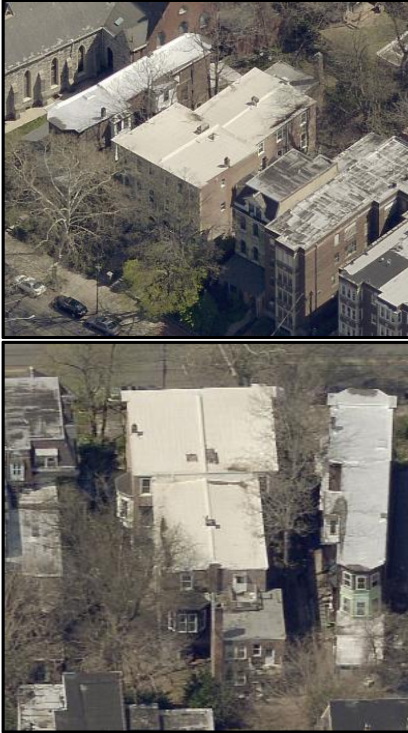
Figure 7. Top: Looking northeast at the primary (west) and south elevations of 405 and 407 S. 42 nd Street. Figure 8. Bottom: Looking west at the rear elevations. Source: Atlas, City of Philadelphia, 2018.
