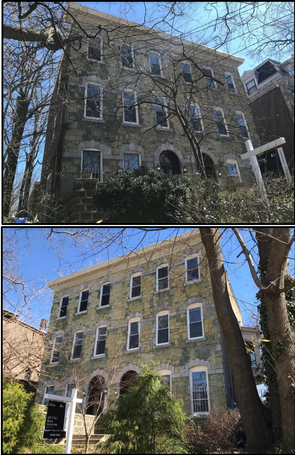
Figure 4. Both photographs show the primary (west) elevation of 405 and 407 S. 42 nd Street. Source: Oscar Beisert, 2019.
