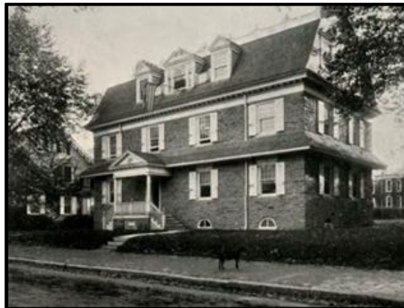
The Colonial Club once stood at the corner of Green Lane and Harvey Street in Germantown. This Colonial Revival style club house was designed as a distinctive building that fit into the suburban context of Germantown and, while it includes many features of the said style, it was a creative, unique work. The Nichols-Goehring House and the Colonial Club both included a pent roof, though the example shown above is more fully articulated. Source: the Germantown Historical Society.
