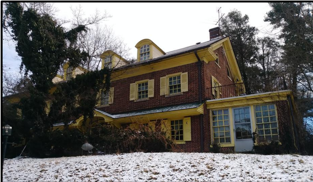
Looking southeast, the John R. Goehring House. Source: Kelly Altrichter.
