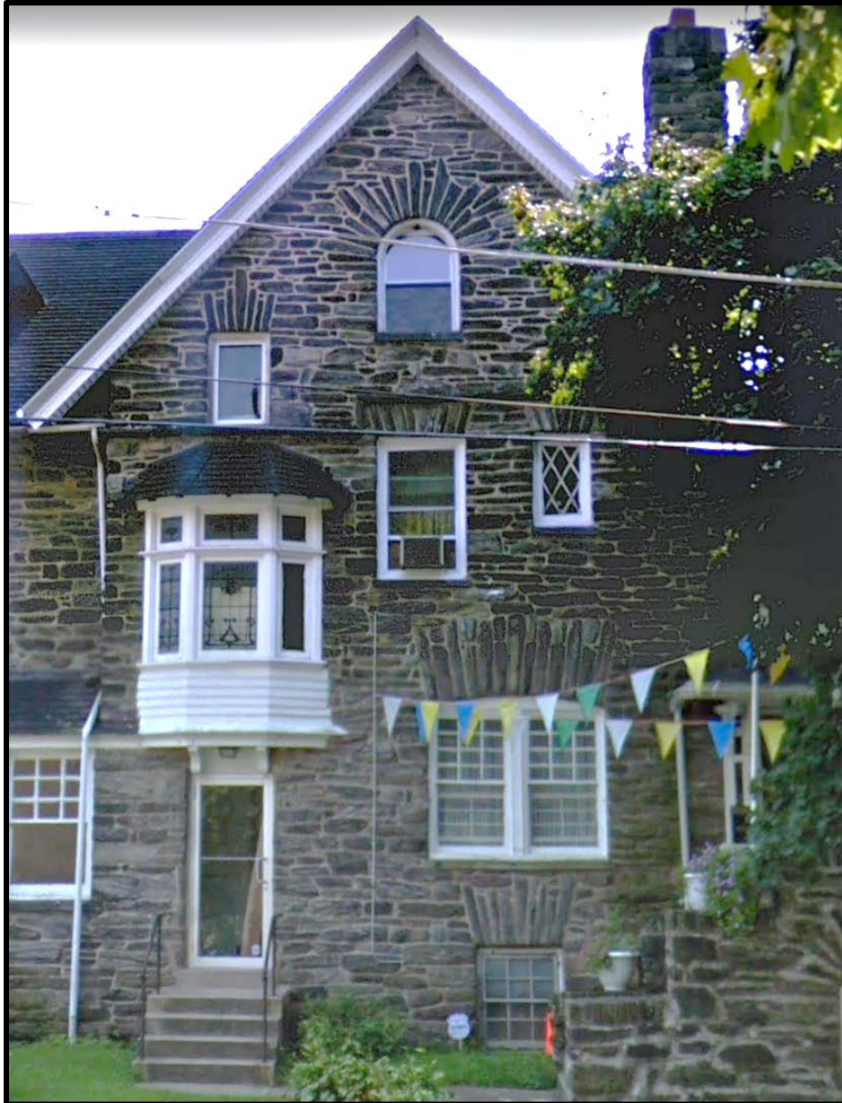
Looking southeast at the side, W. Phil Ellena Street elevation of the primary elevation. Source: Google, 2018.
