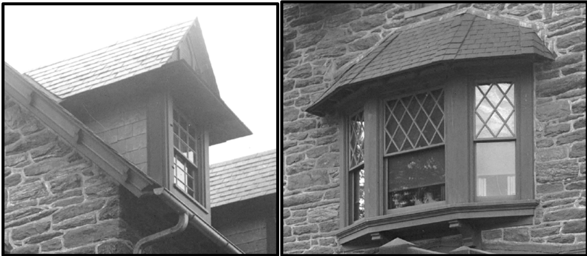
Left: Detail of a photograph taken by Franklin Davenport Edmunds (1874–1948) of a gable-front dormer window within the side, W. Phil Ellena Street elevation of the subject property in 1909. Right: Detail of a photograph taken by Franklin Davenport Edmunds (1874–1948) of a bay window within the primary elevation of the subject property in 1909. Source: Digital Collections of the Free Library of Philadelphia, 2018.
