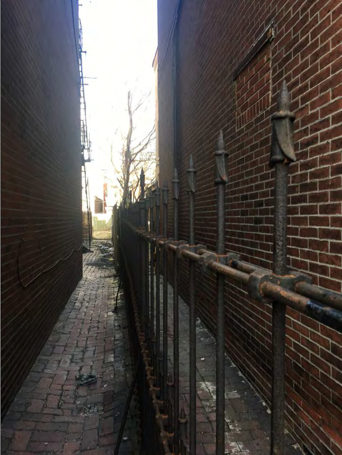
Figure 8. Detail of cast-iron fence between 713 and 715 N. 6 th Streets. Photo taken by Arielle Harris, April 2018.
