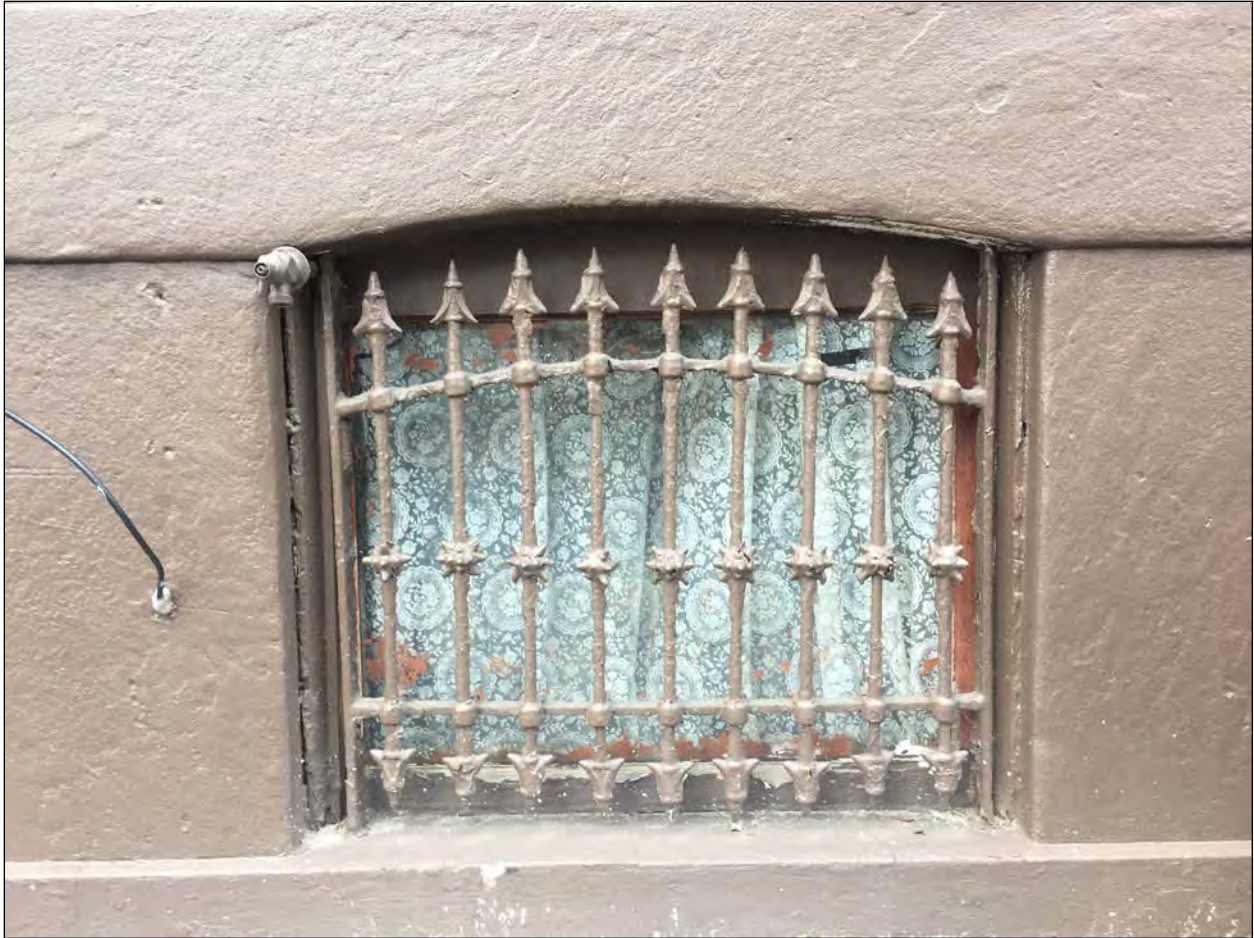
Figure 8. Detail of cast-iron ground floor window bars at 713 N. 6 th Street. Photo taken by Arielle Harris, April 2018.
