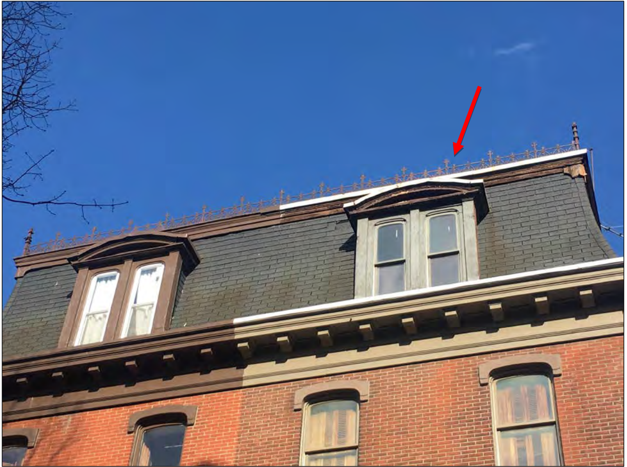
Figure 9. Detail of cornice and cast iron cresting at 711-713 N. 6 th Street. Photo taken by Arielle Harris, April 2018.
