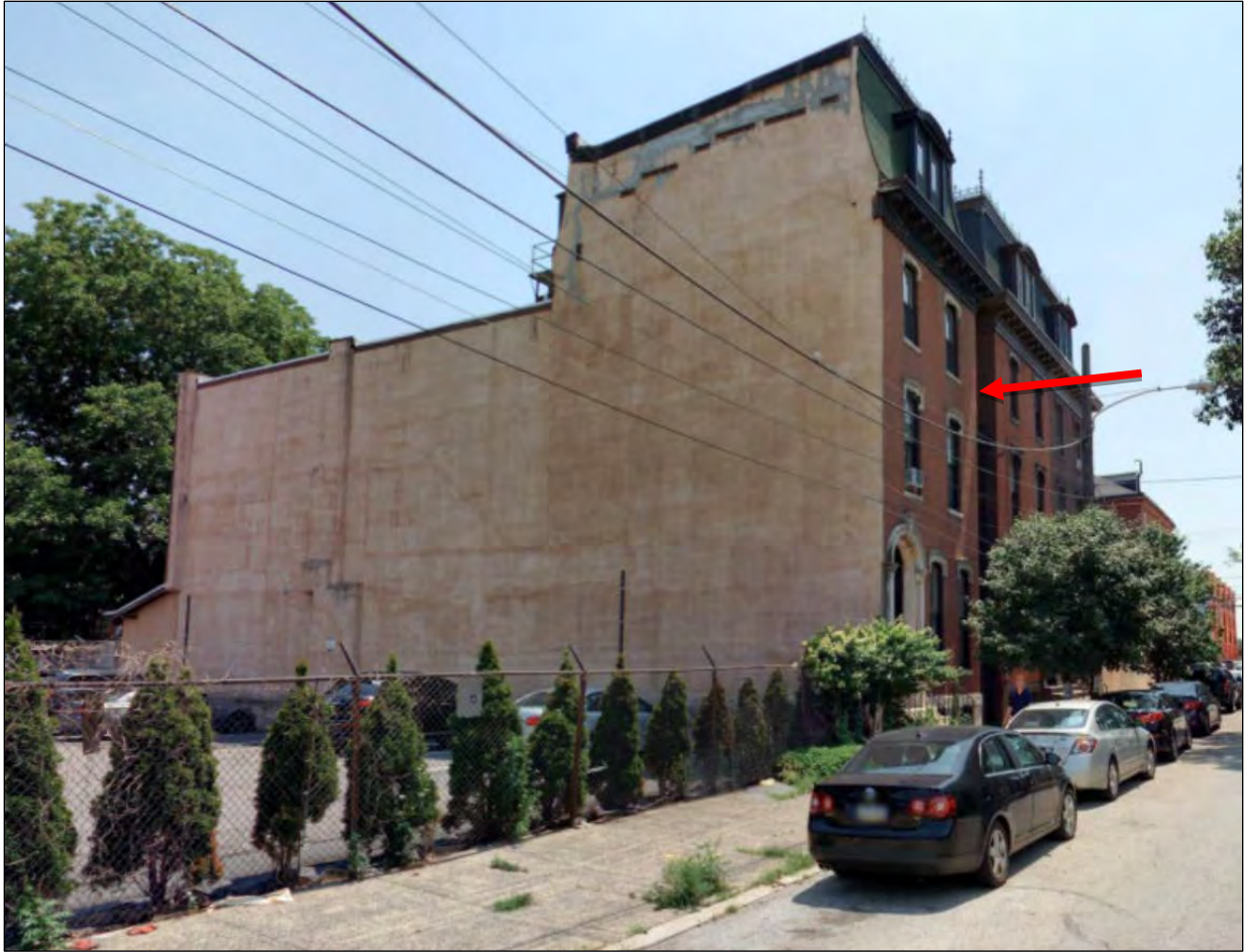
Figure 6. Looking south down 6 th Street. 715 N. 6 th Street is indicated by the red arrow. Cyclomedia, July 2018.
