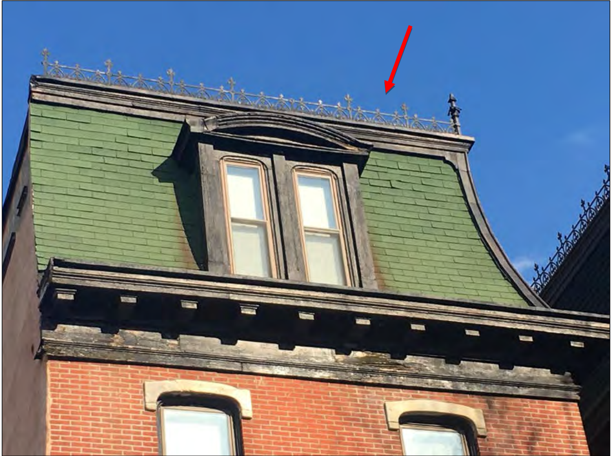
Figure 8. Detail of cornice and cast iron cresting at 715 N. 6 th Street. Photo taken by Arielle Harris, April 2018.
