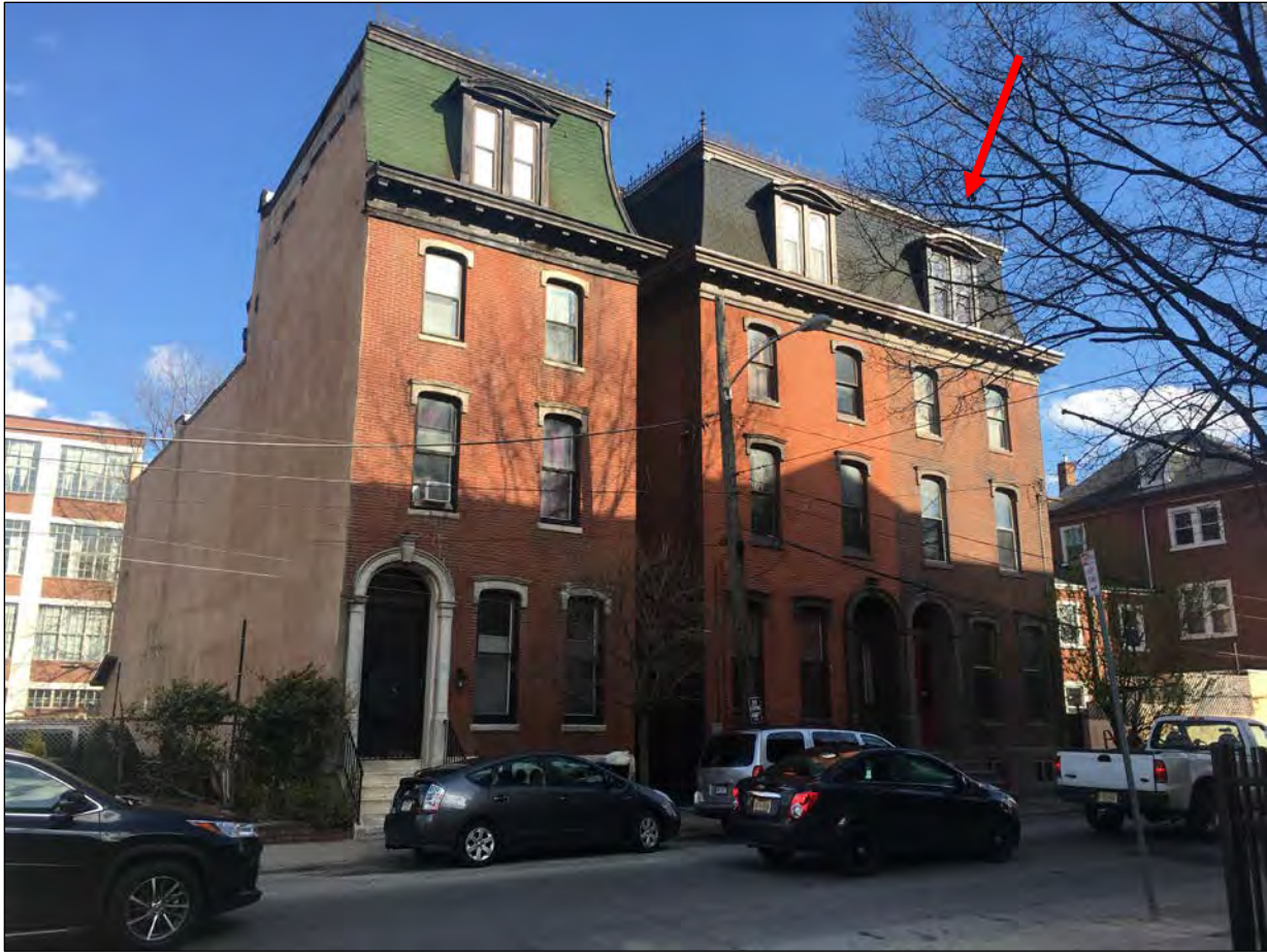
Figure 4. 711-715 N. 6 th Street. 711 is at the right. Photo taken by Arielle Harris, April 2018.
