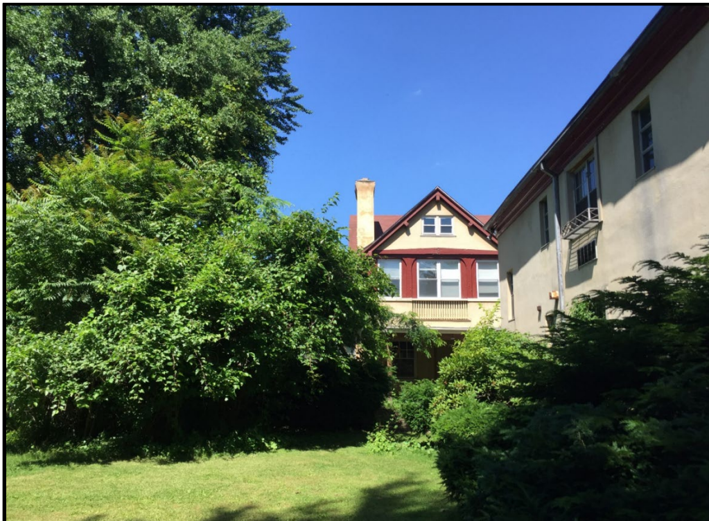
Photo No. 34: Looking northeast at the rear elevation of the house. Source: Keeping Philadelphia, 2018.
