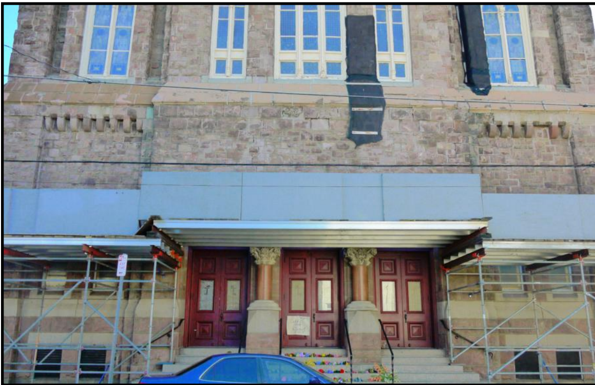
Looking southwest, the first stage of the primary elevation.
