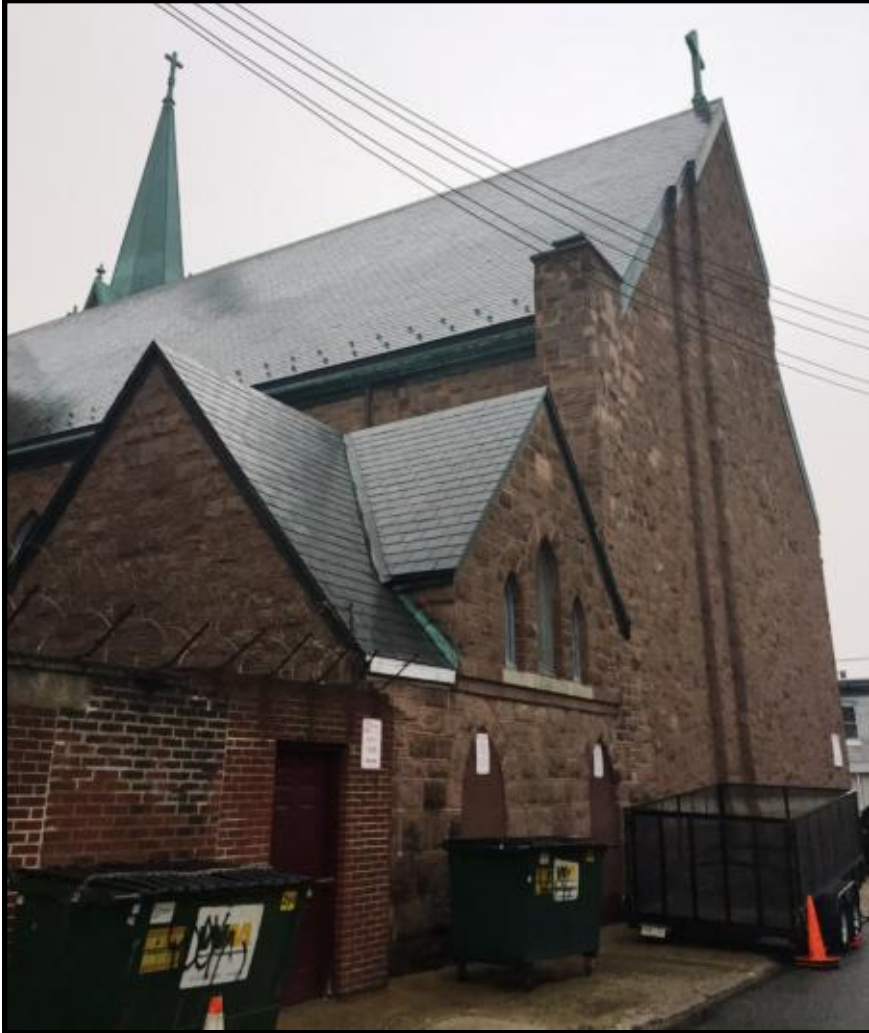
Looking northeast, the rear elevation of the ell and the church.
