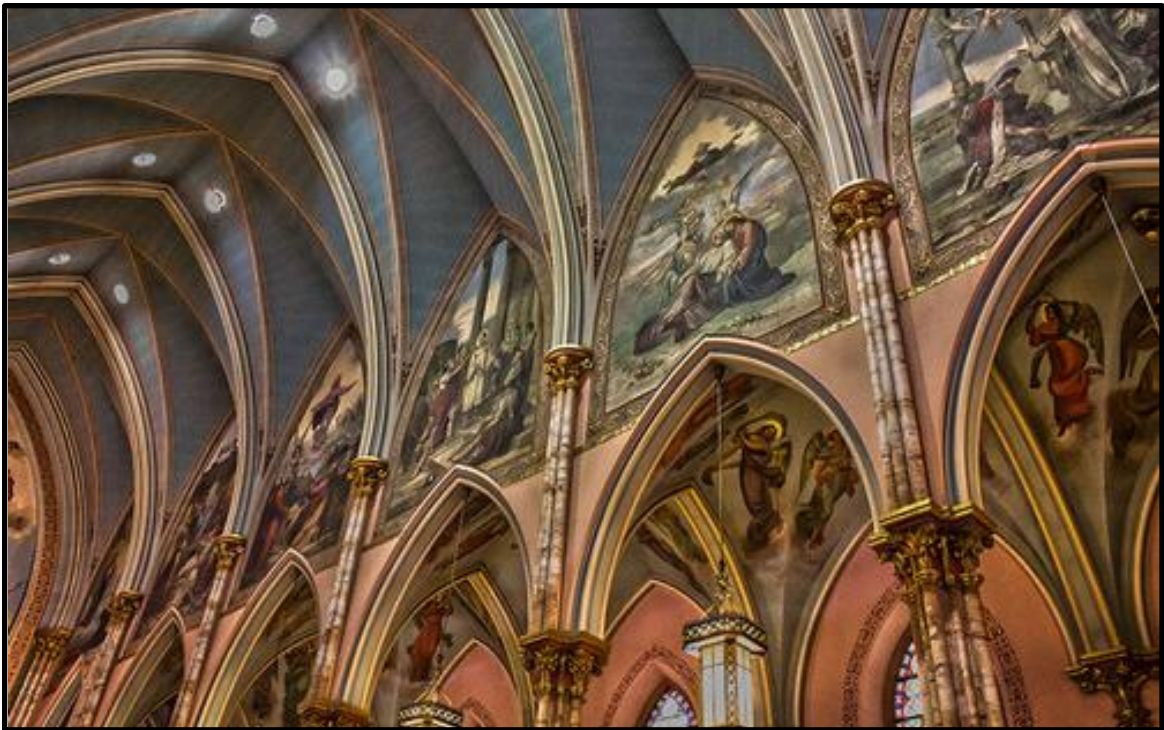
The ceiling and aisle of St. Laurentius Church.
