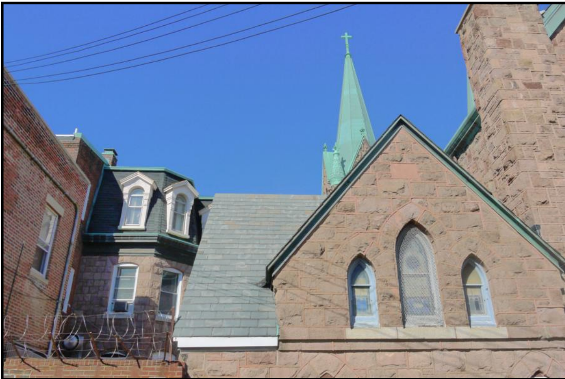
Looking north, the rear, south elevation of the rectory and church.
