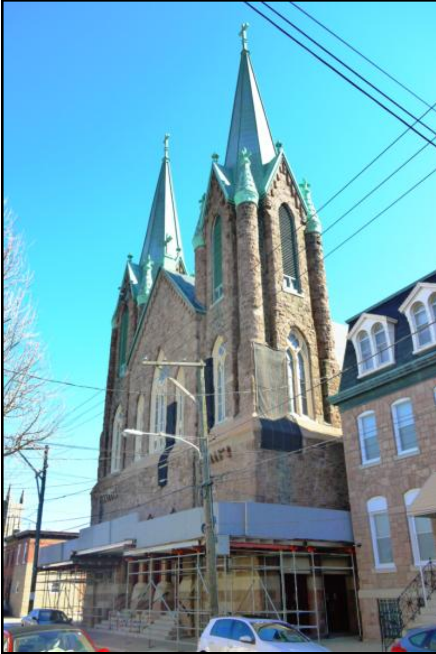
Looking southeast, the primary and northwest elevation of the church.
