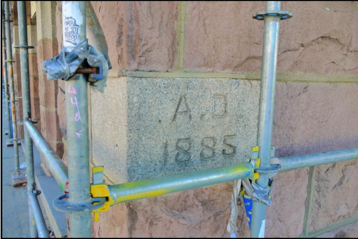
Looking southwest, the cornerstone dating to construction of the basement in 1885.
