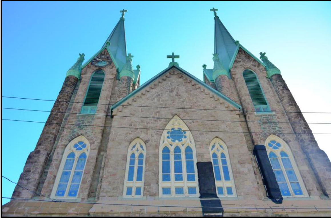
Looking southwest, the upper stages of the primary elevation.
