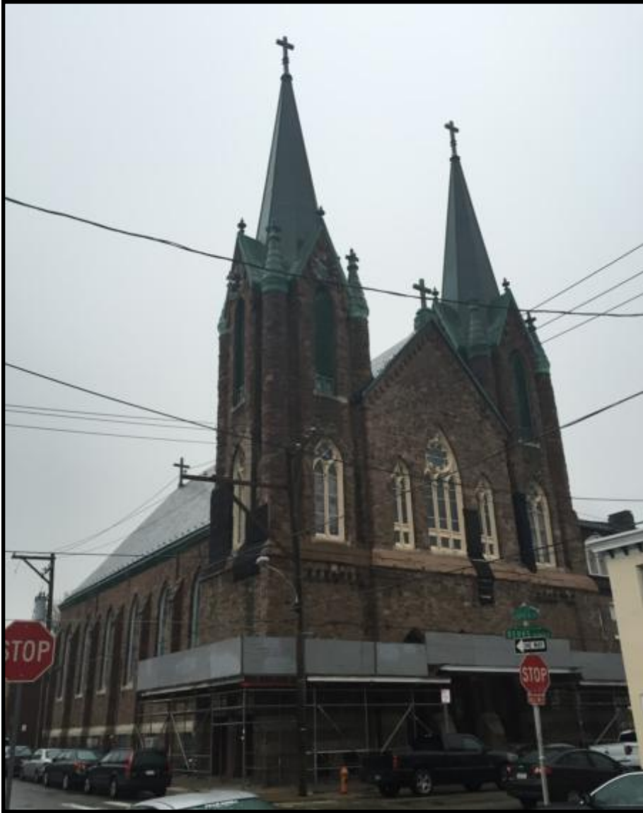
Looking southwest, the primary elevation of the church.
